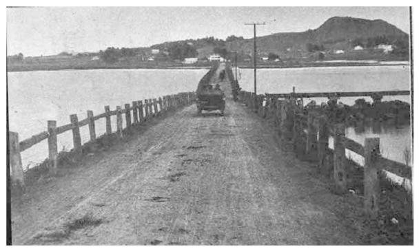
**Figure 21:** View from Onehunga towards Māngere, showing a car crossing to Māngere, 1913. Both ends of the bridge are on causeways, which are linked by the bridge and may date from the 1875 bridge. Sir George Grey Special Collections, Auckland Libraries, 7-A2945.
