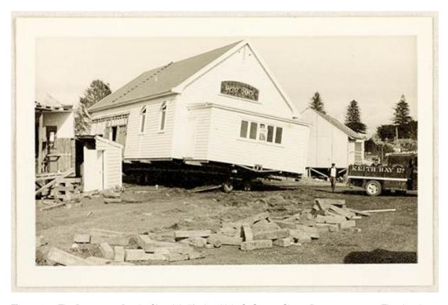
**Figure 186:** The Papatoetoe Baptist Church is lifted on high, St George Street, Papatoetoe, 1970. The church, which had been opened in 1934, was being moved back on the site to make way for a new church (both buildings have since been demolished) (Auckland Libraries Footprints 05422).
