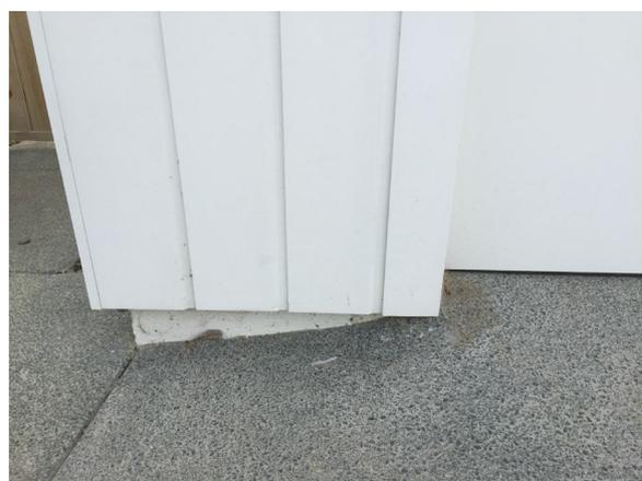
E2/AS1 compliant ground clearance at garage door
