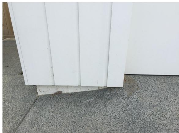
E2/AS1 compliant ground clearance at garage door
