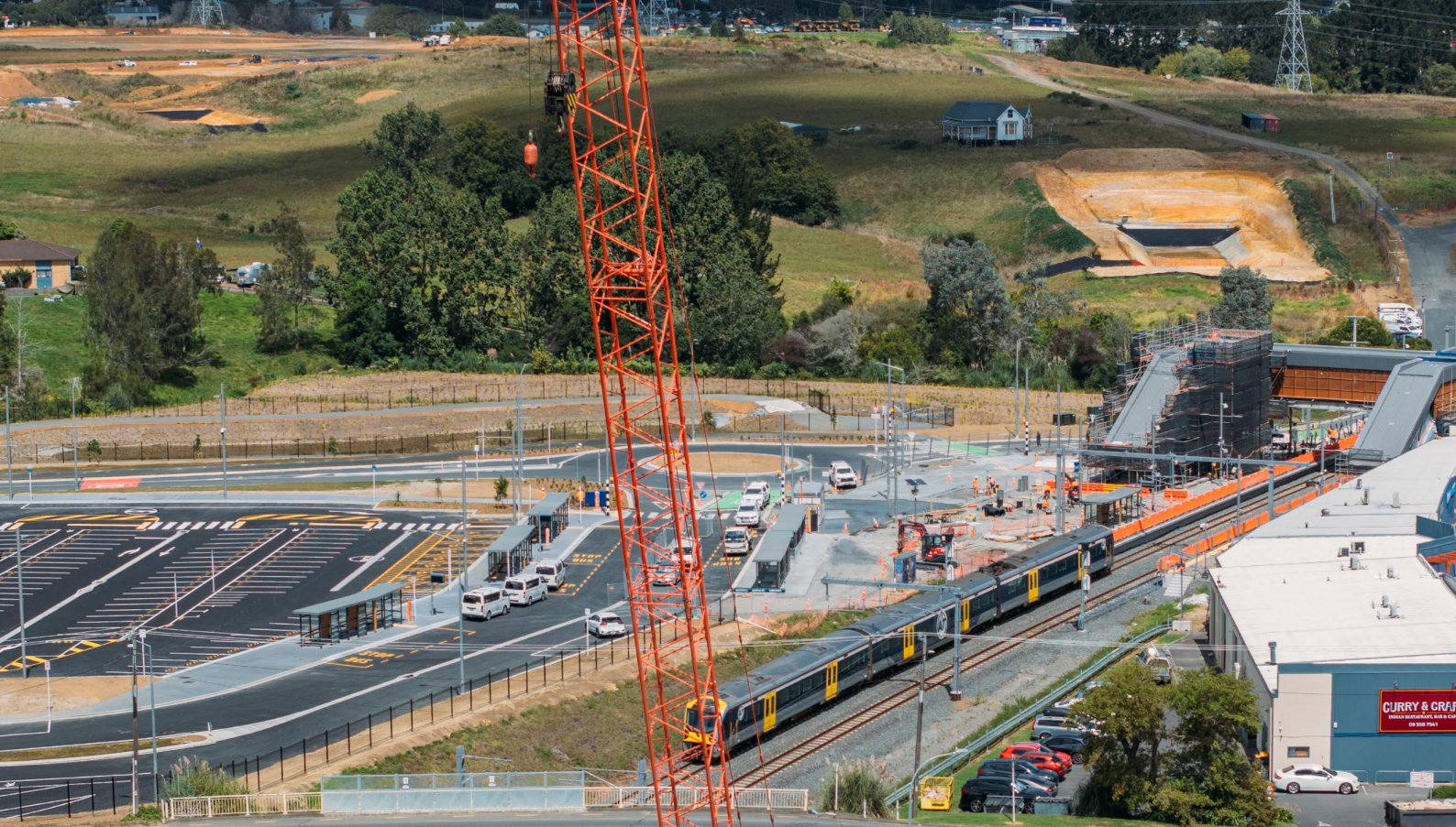
Under construction: Drury takes shape as a future-ready urban development area.
