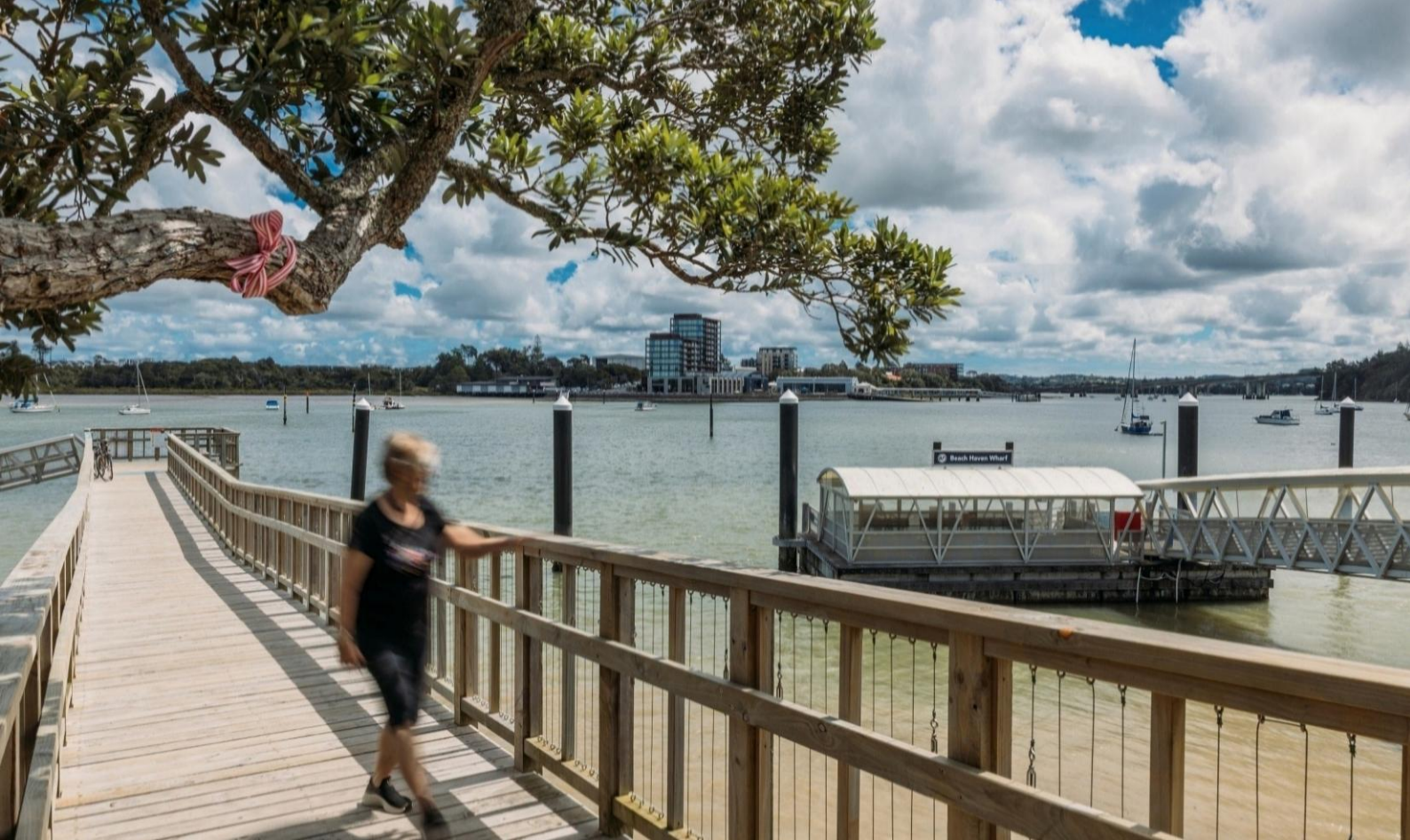
Beach Haven ferry terminal.
