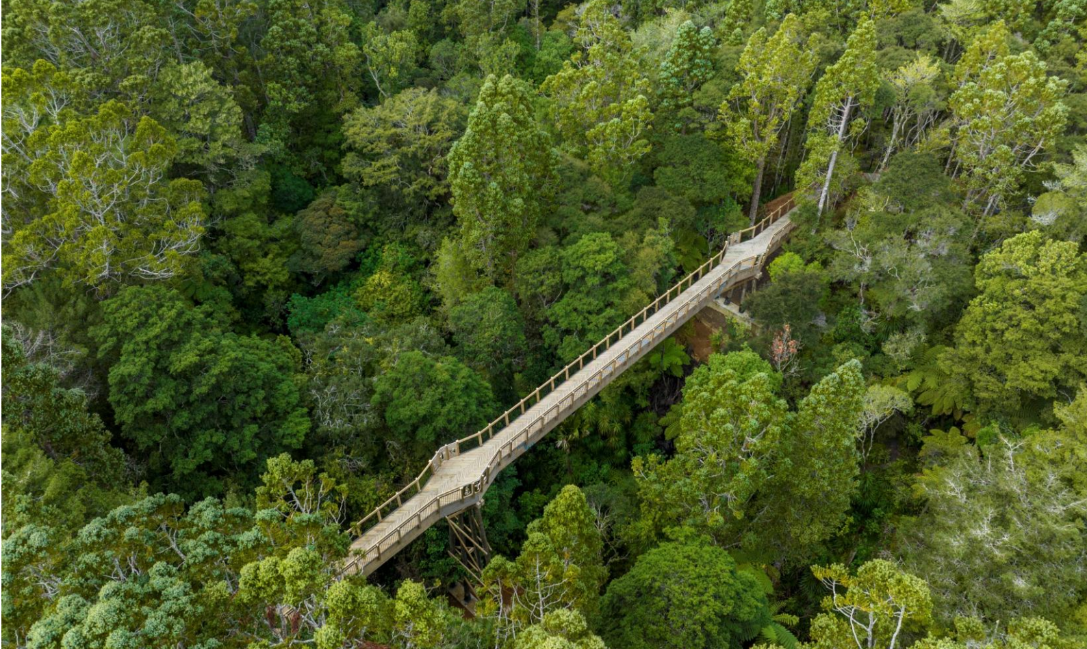
The bridge at Kauri Glen Reserve offers views of mature forest canopy while helping prevent the spread of kauri dieback.
