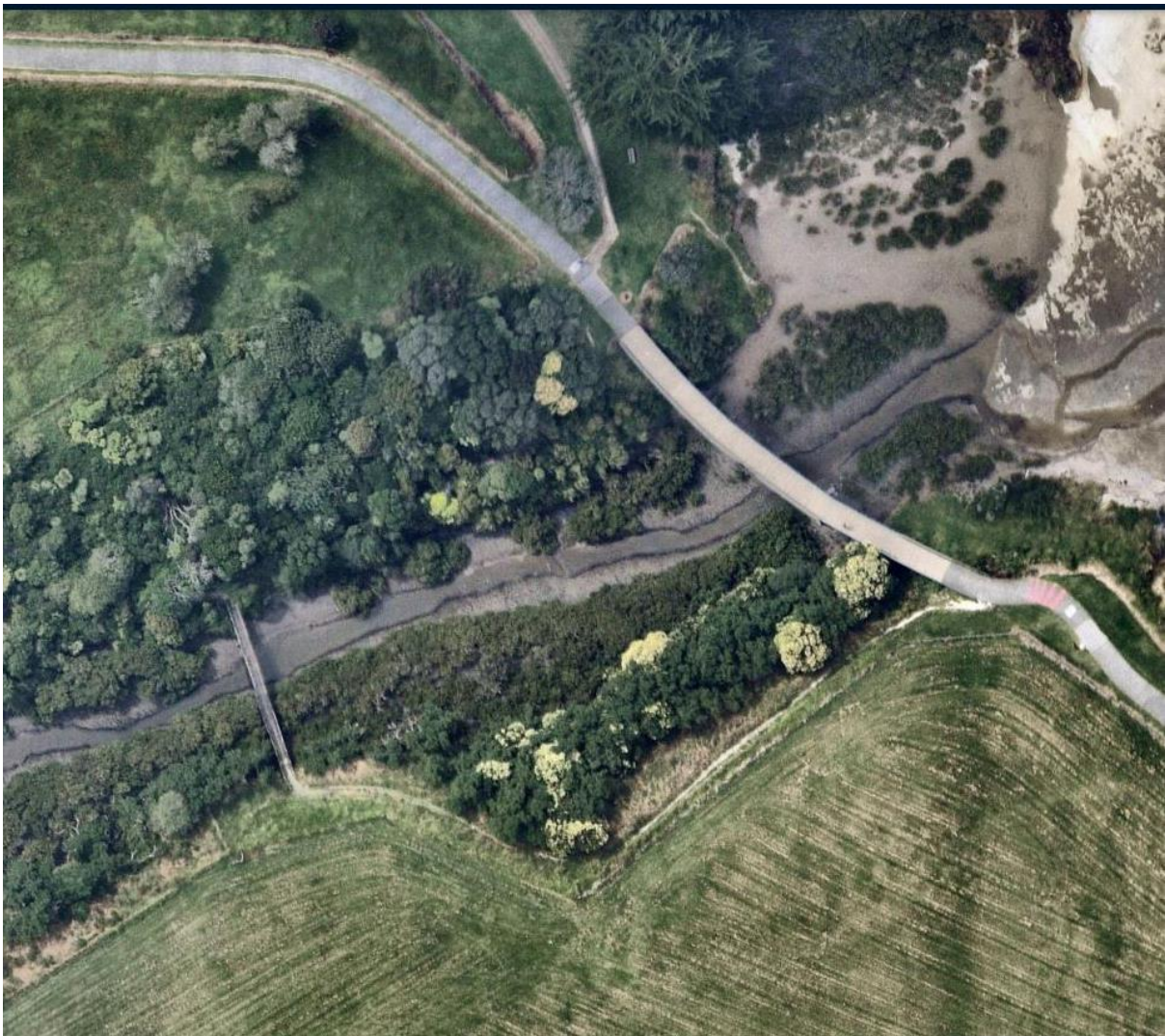
Image 2: existing bridge shown to the west, new bridge to the east (completed 2021)
