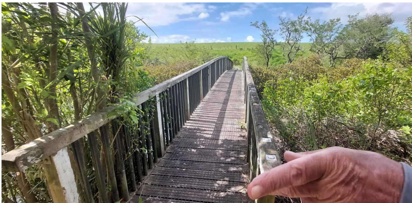
Image 3: existing bridge to be decommissioned.
