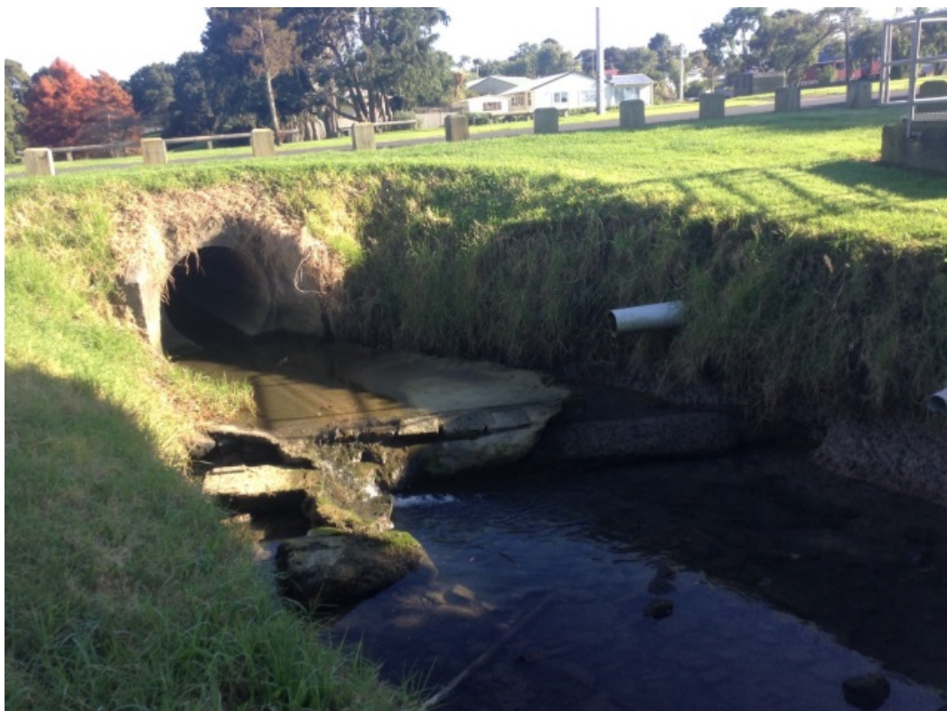
Figure 7: Culvert and concrete apron below Riverside Road
