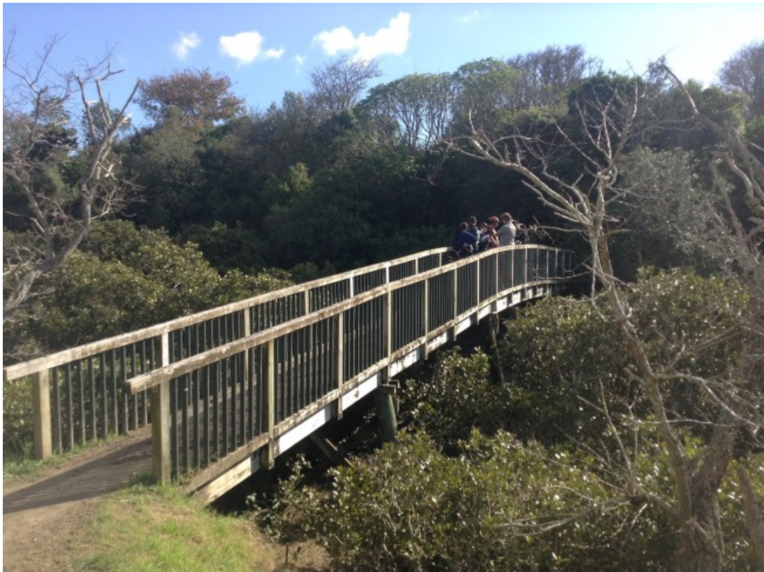
Figure 5: Existing bridge across Omaru Creek
