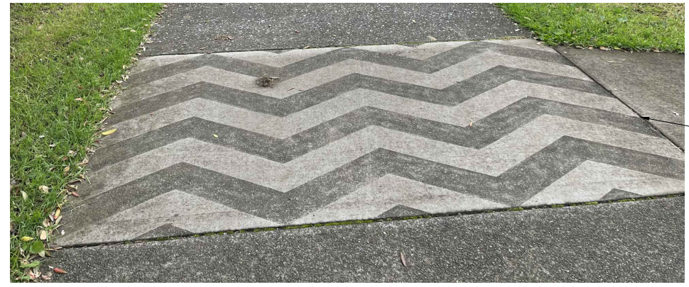
3 - SAND BLASTED 'ZIGZAG' MOTIF DETAIL NTS
