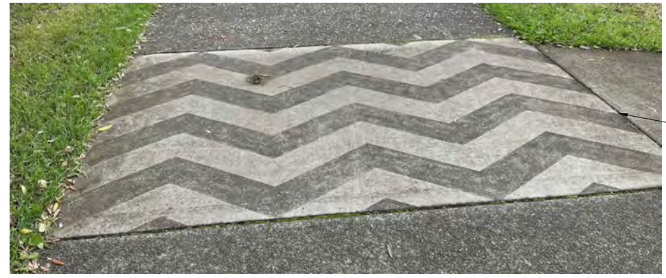
3 SAND BLASTED 'ZIGZAG' MOTIF DETAIL NTS
