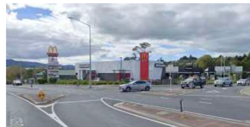
Photo Source: Google Maps The Grange convenience retail complex located on State Highway 1
