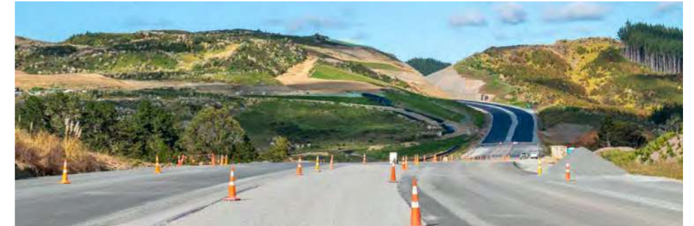
Photo Source: www.nzta.govt.nz Puhoi to Warkworth motorway
