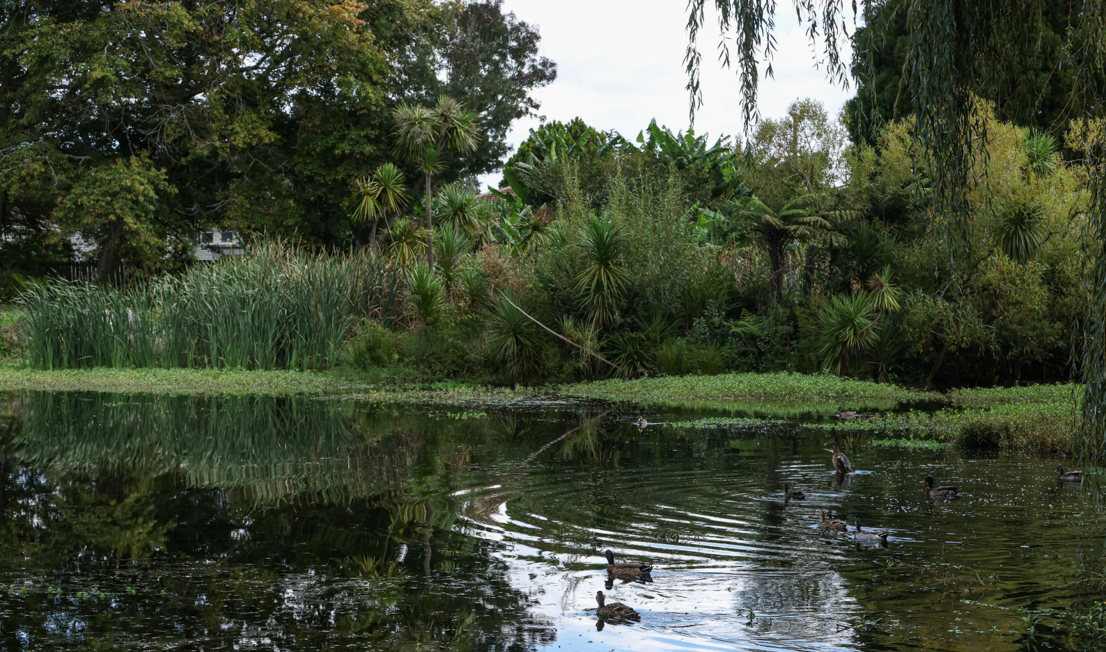
Te Koiwi stormwater pond designed to reduce downstream flooding, improve water quality and mitigate erosion by capturing stormwater when it rains.
