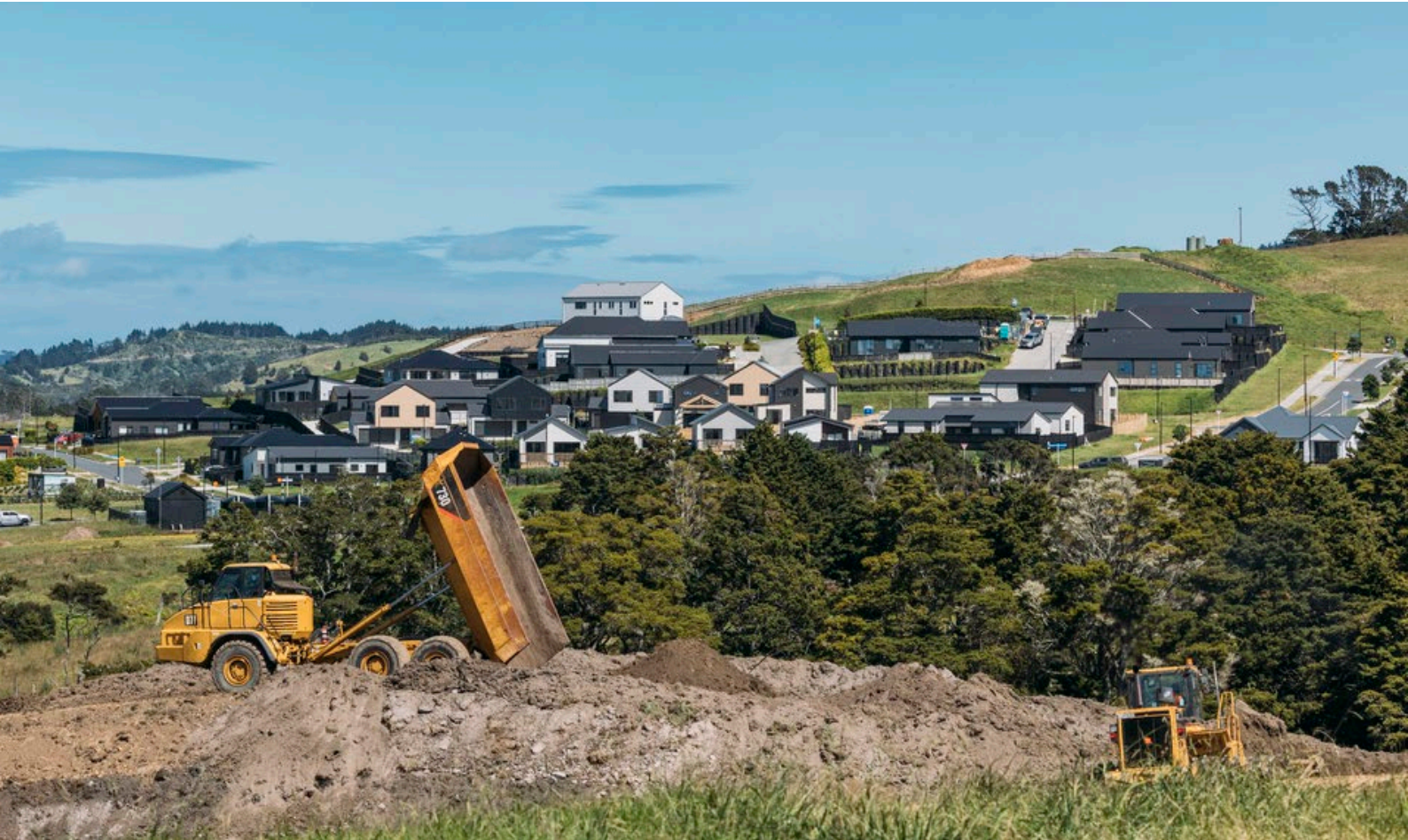
Construction is underway at a new development in Warkworth.
