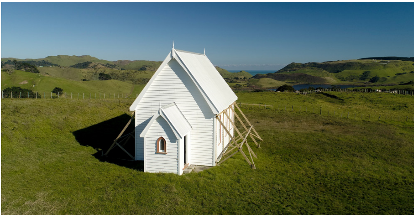
Image: The Kohekohe Church before its adaptive reuse. Temporary supports were placed to stabilise the building due to the imminent risk of collapse (Photograph courtesy of Guy Quartermain, April 2021).
