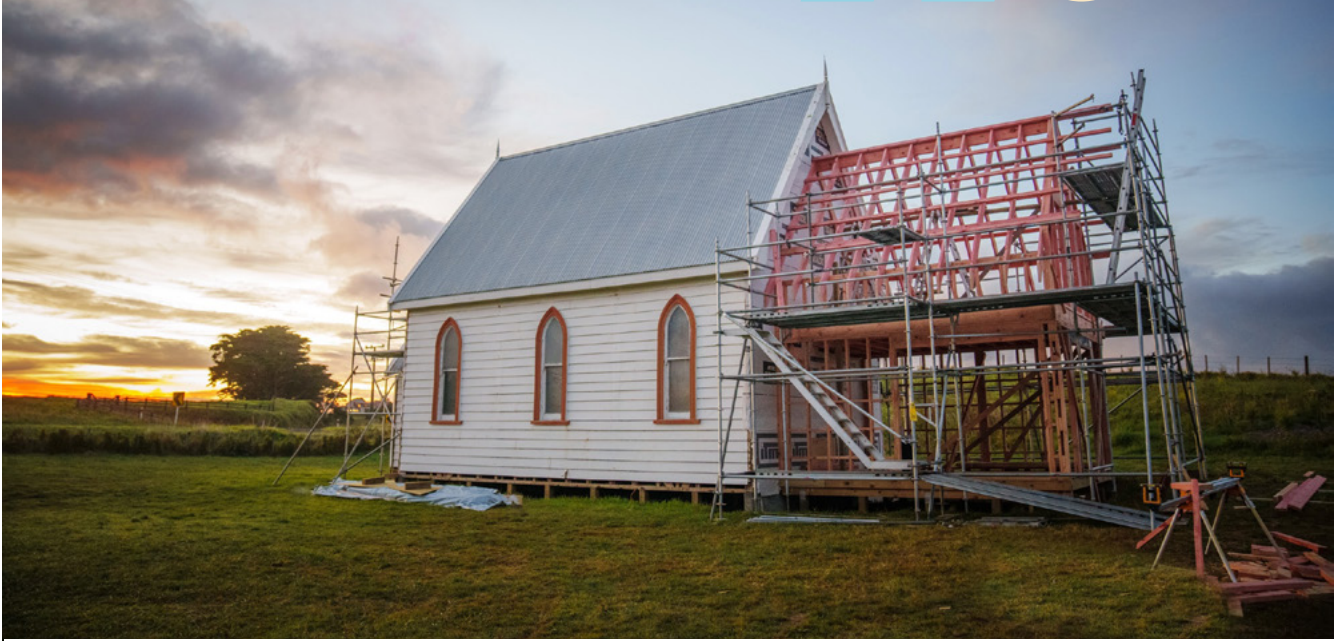
Image: During the construction of the addition (photograph courtesy of Guy Quartermain, February 2024).
