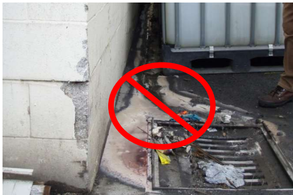
Keep chemicals away from stormwater drains
