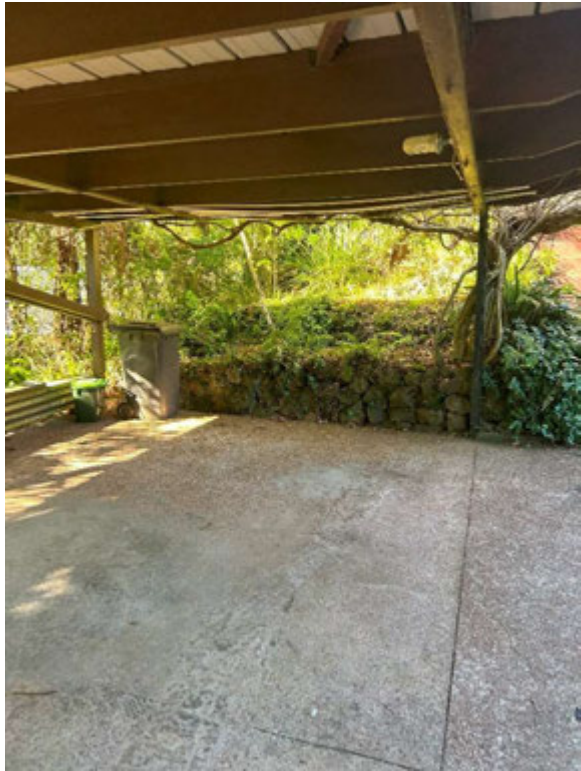
Picture 2: Existing Carport
