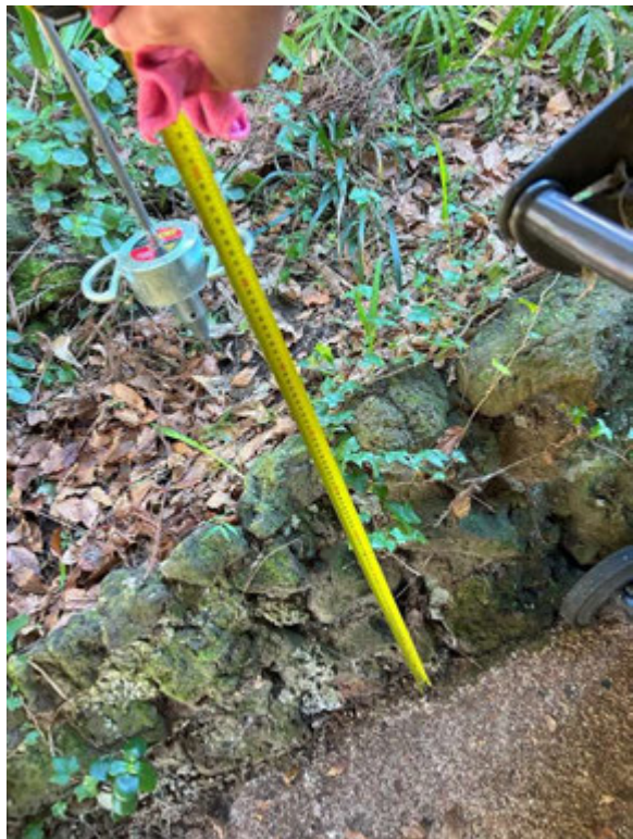
Picture 39: Scala 3 Test Area near Carport
