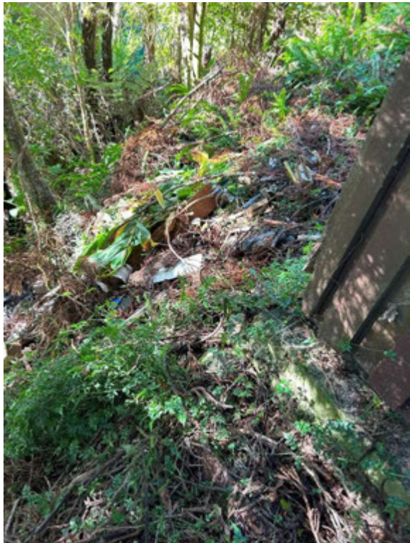
Picture 8: Existing Shed Foundation Edge near Slope
