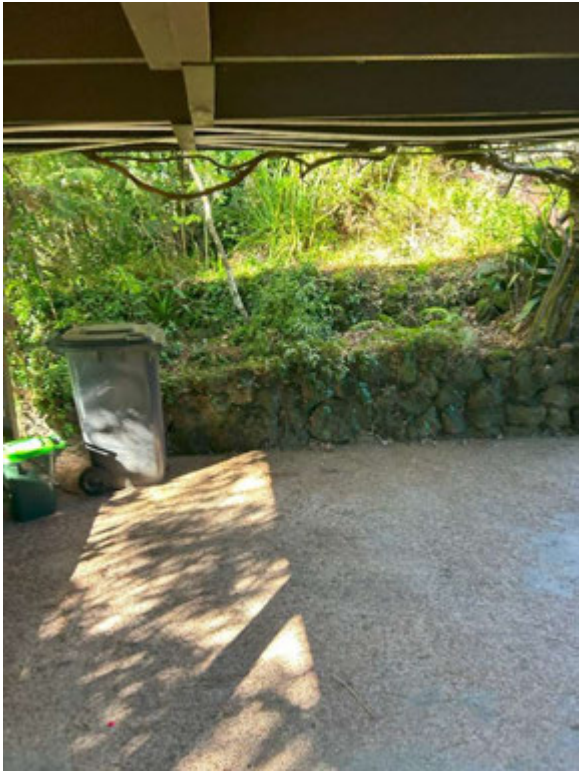
Picture 1: Existing Carport before Removal
