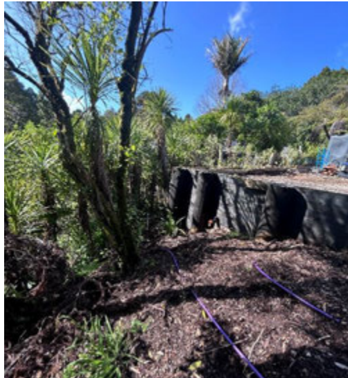
Picture 12: Timber retaining wall by garage (2)
