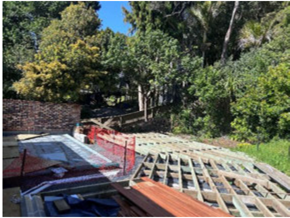
Picture 4: Decking area (2)
