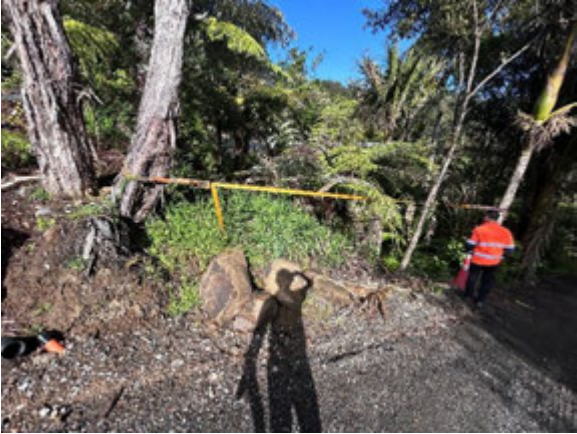
Picture 9: Higher tank stormwater overflow area
