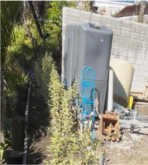
Picture 11: Lower Tank not yet in place
