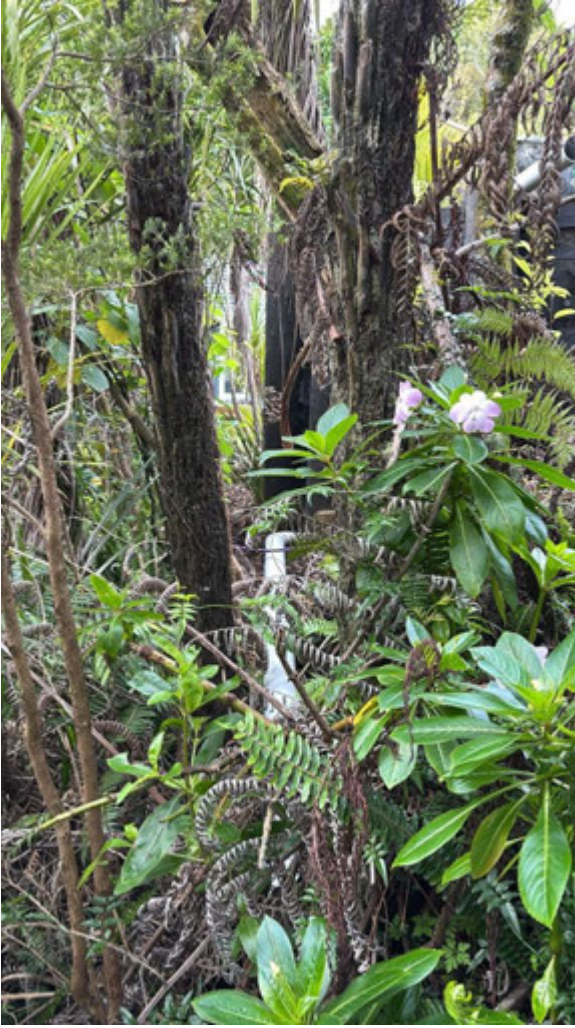
Picture 21: 3 Subsoil pipe extensions into dense vegetation
