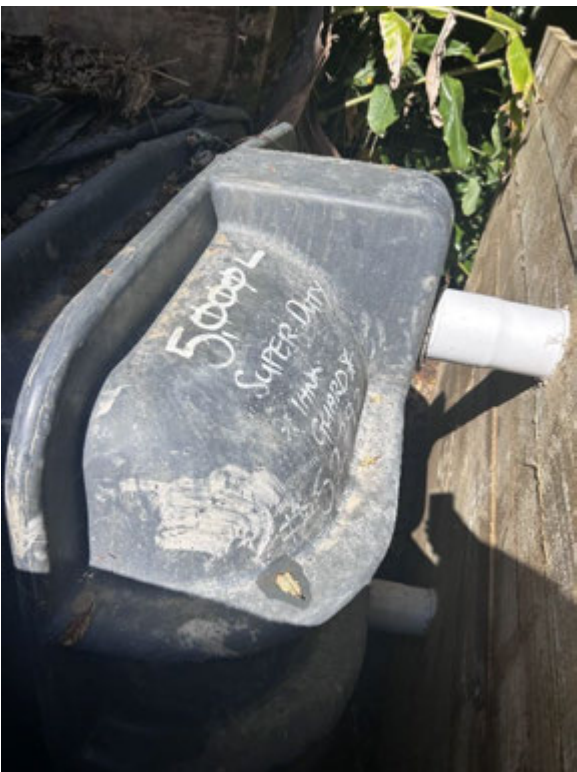
Picture 7: Higher Tank in Place but not backfilled
