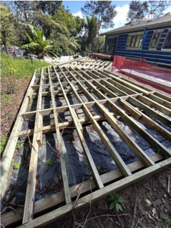
Picture 5: Decking area
