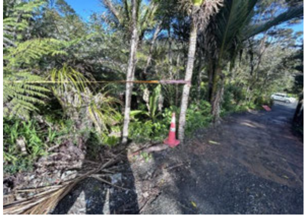
Picture 10: Lower Overflow area
