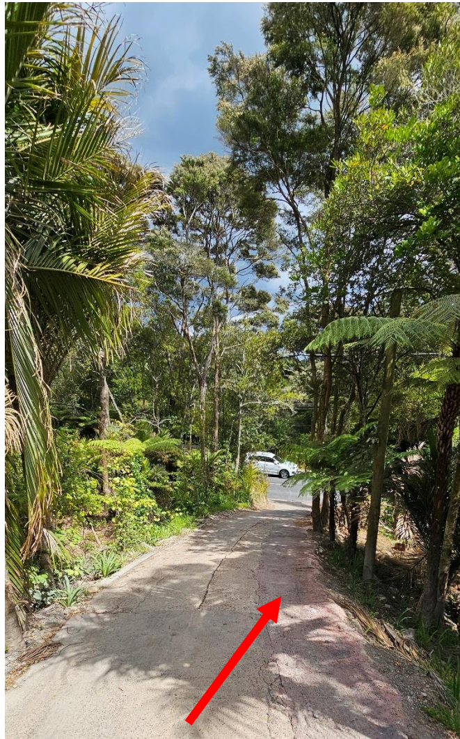
Figure 4: Visible signs of driveway widening (arrow)
