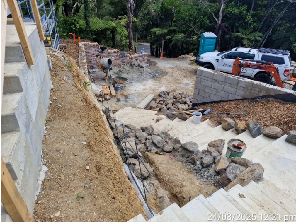
Figure 1: from main dwelling, looking down driveway to Konini Road
