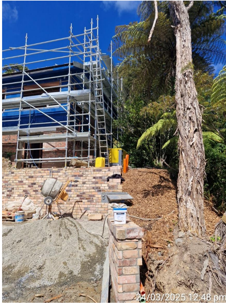
Figure 5: looking retaining wall of main dwelling.
