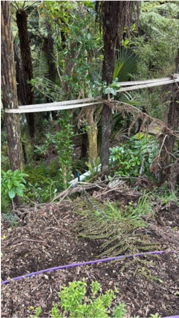
Picture 19: 3 Subsoil pipe extensions into dense vegetation (2)
