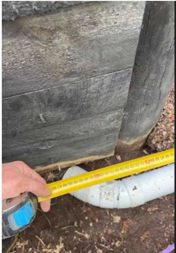
Picture 18: 2 Subsoil Outlet Connected
