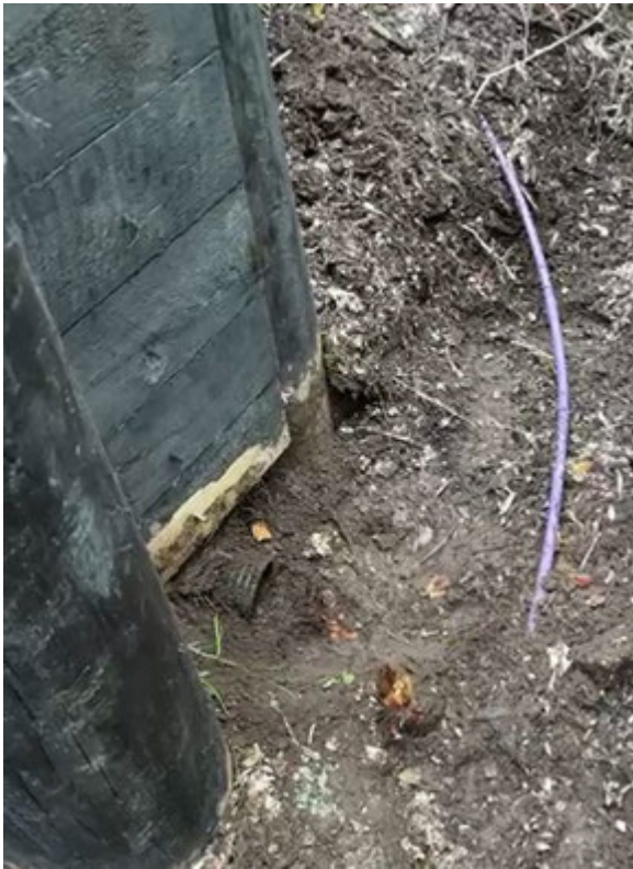
Picture 17: 1 Subsoil Outlet Exposed
