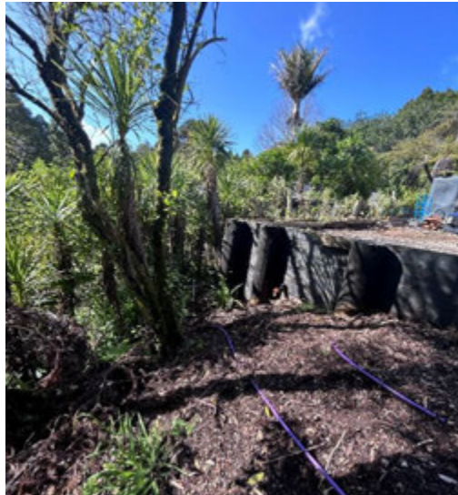
Picture 12: Timber retaining wall by garage (2)
