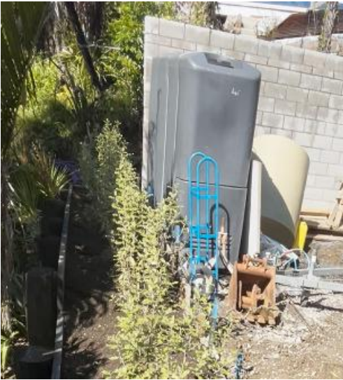
Picture 11: Lower Tank not yet in place
