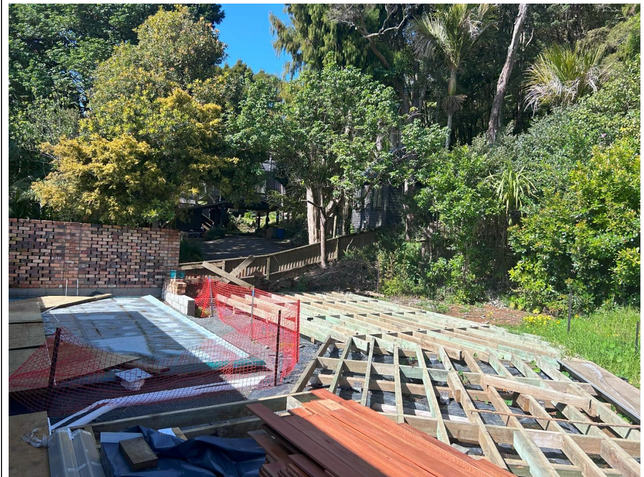
Figure 6: Photo showing current Construction/Proposed Layout
