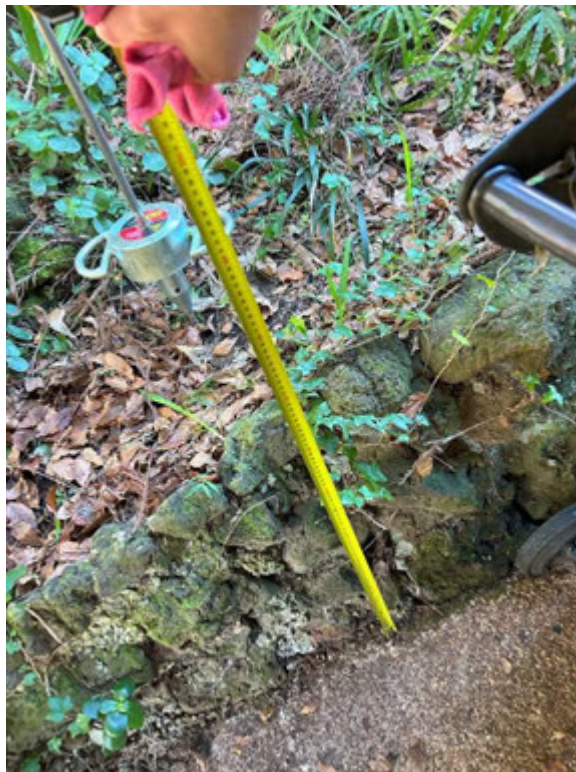
Picture 39: Scala 3 Test Area near Carport
