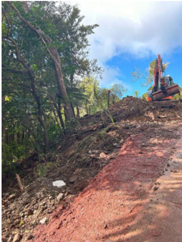
Picture 4: Existing Driveway Being Extended
