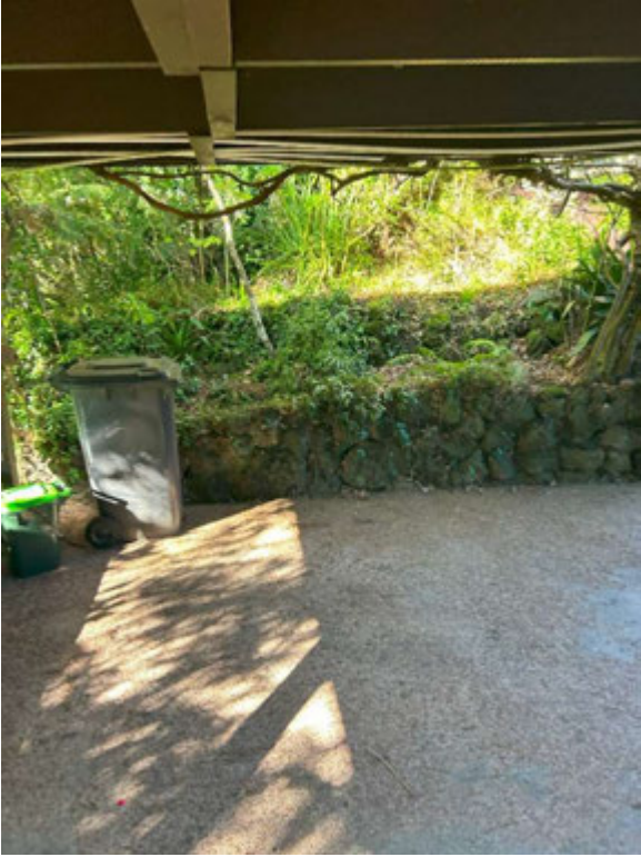
Picture 1: Existing Carport before Removal
