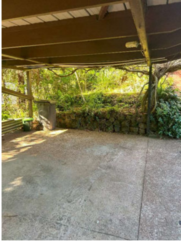
Picture 2: Existing Carport
