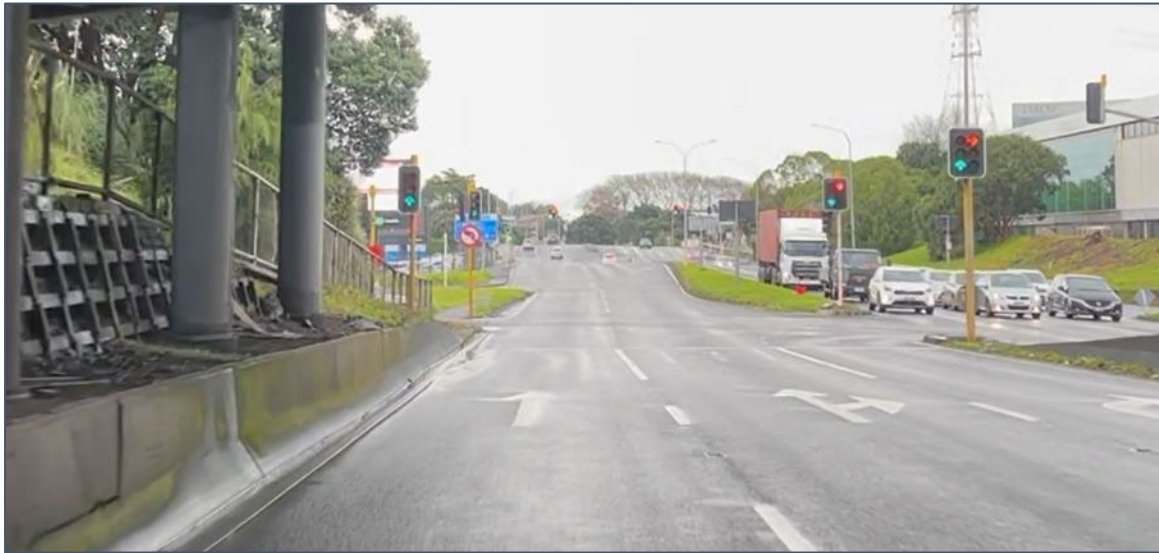
Figure 8: Lane 1 commencement of plan view visual overlap (~40.5m from limit line)
