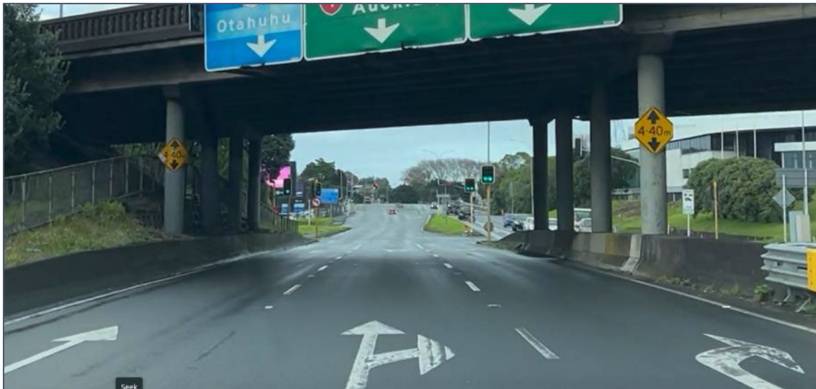
Figure 12: Lane 2 commencement of plan view visual overlap (~78m from limit line)
