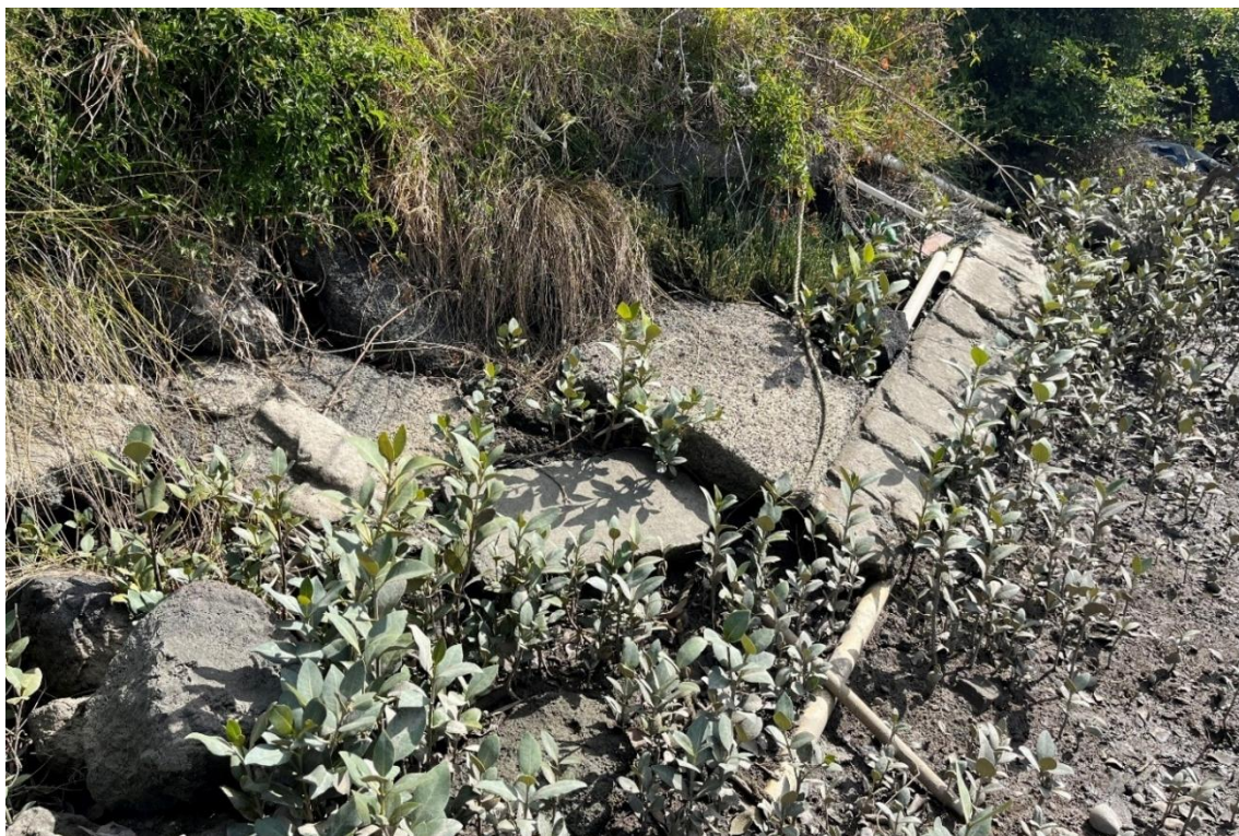
Figure 6: Informal armoring structures at the toe of the slope (149 Edgewater Drive).
