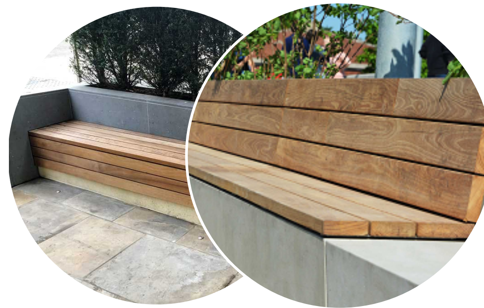
Recessed timber seating on retaining wall
