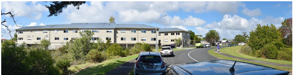
Figure 4: View of the Site looking south down Edgewater Drive
