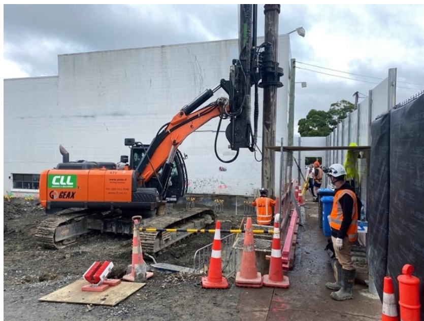
Figure 7 - Example of augering with attachment on short reach 13T excavator boom
