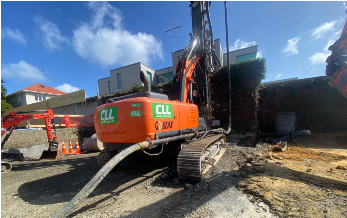
Figure 5 – 78T CFA rig (58T Crawler) operating adjacent a boundary
