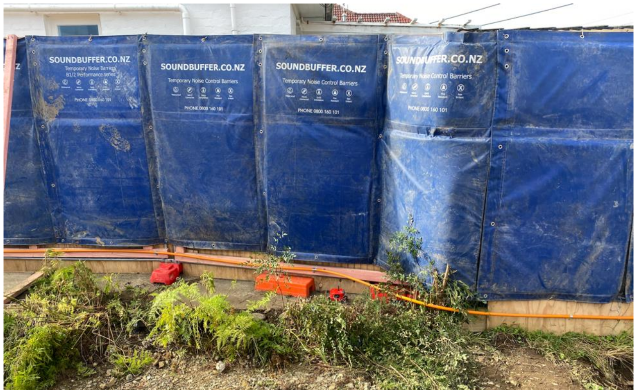
Figure 16 - Example of Acoustic blankets affixed to existing landscape fences
