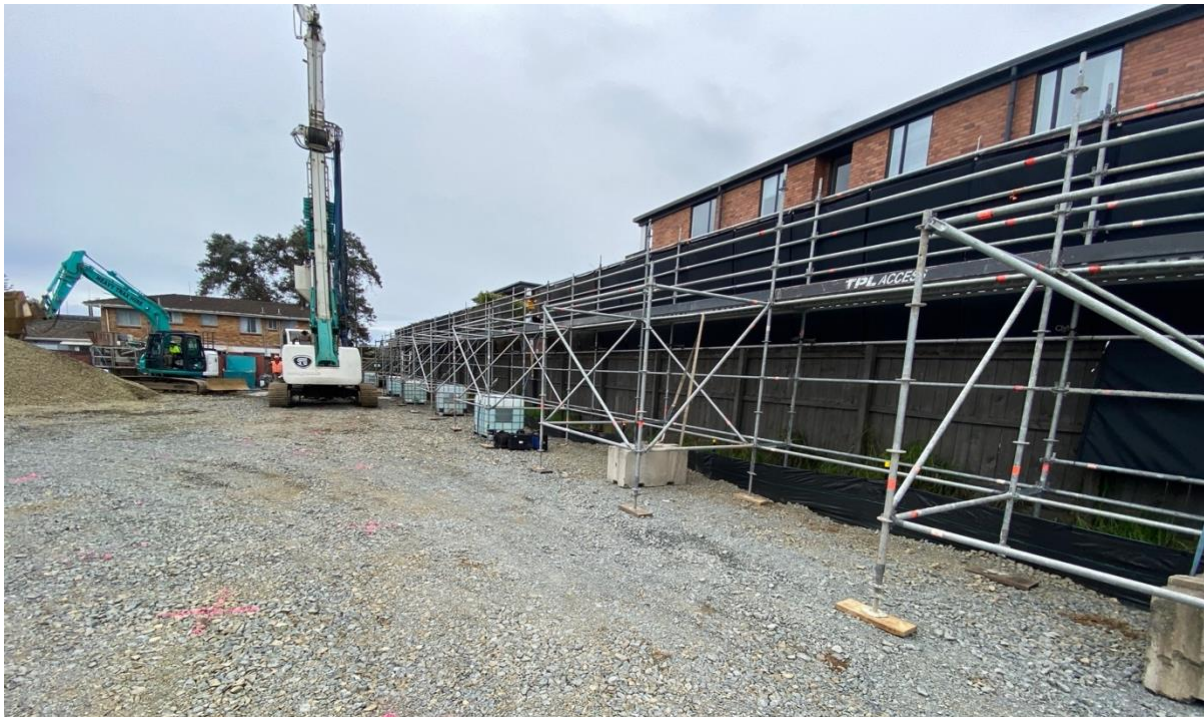
Figure 20 – 4m-6m Acoustic Blankets on Scaffolding
