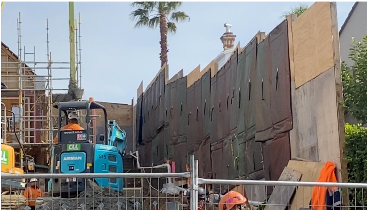
Figure 12 - 4m Plywood Fence with acoustic blanket lining
