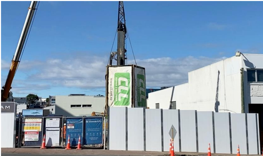
Figure 21 - Hoisted Shielding Example
