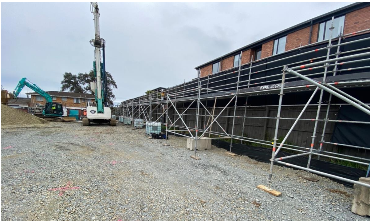
Figure 14 – 4m-6m Acoustic Blankets on Scaffolding
