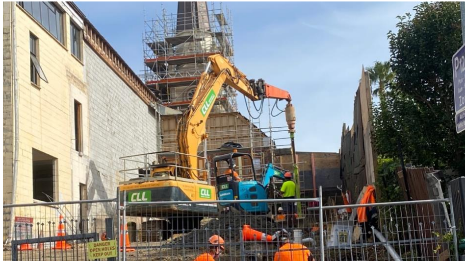
Figure 6 - Example of Augering with attachment on long reach 23T excavator boom
