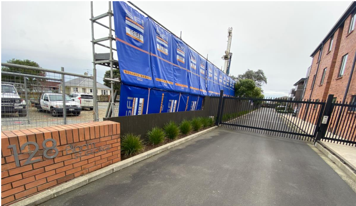
Figure 19 – 4m-6m Acoustic Blankets on Scaffolding
