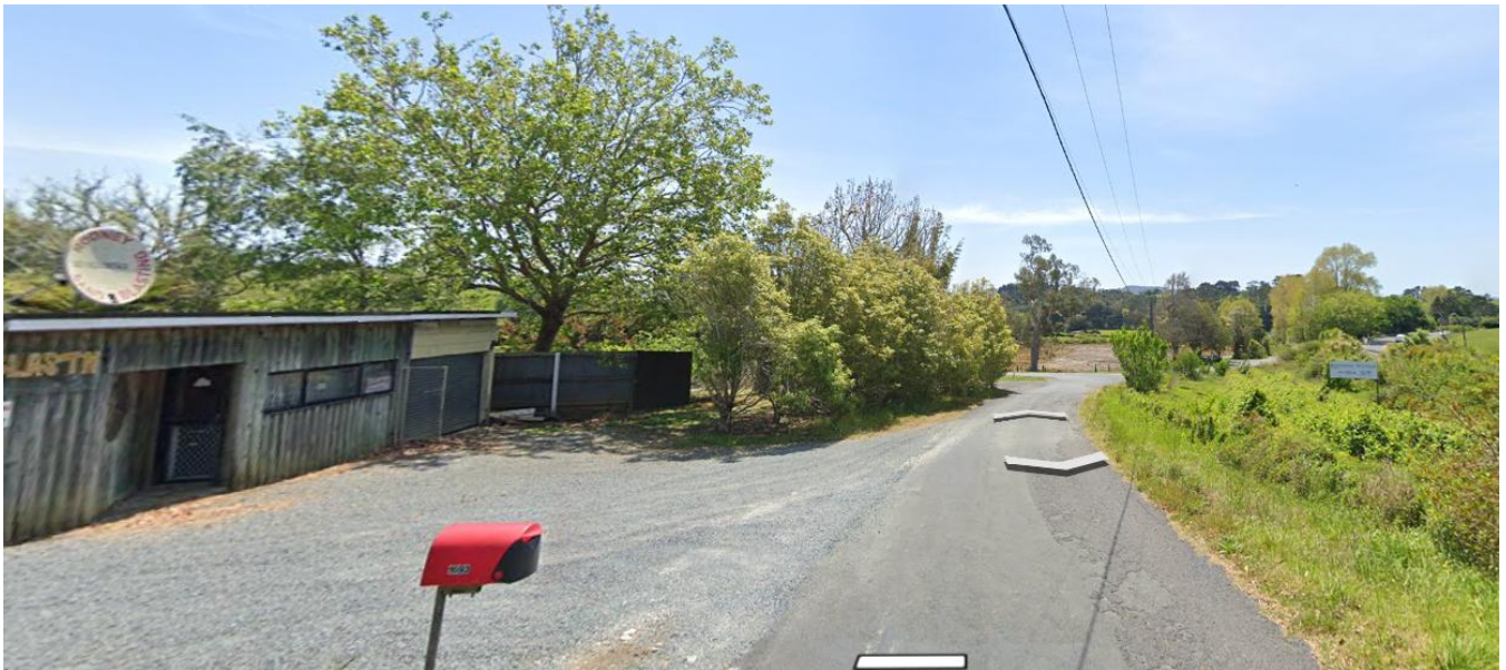
Figure Seventeen: Valerie Close with New Vehicle Crossing Location Just Past End of Shed.
