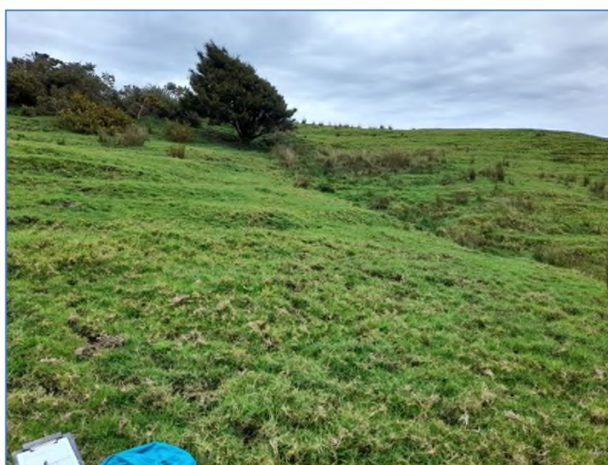
Figure 2: Example of observed historic landslide morphology northeast of the proposed Lot 8.
