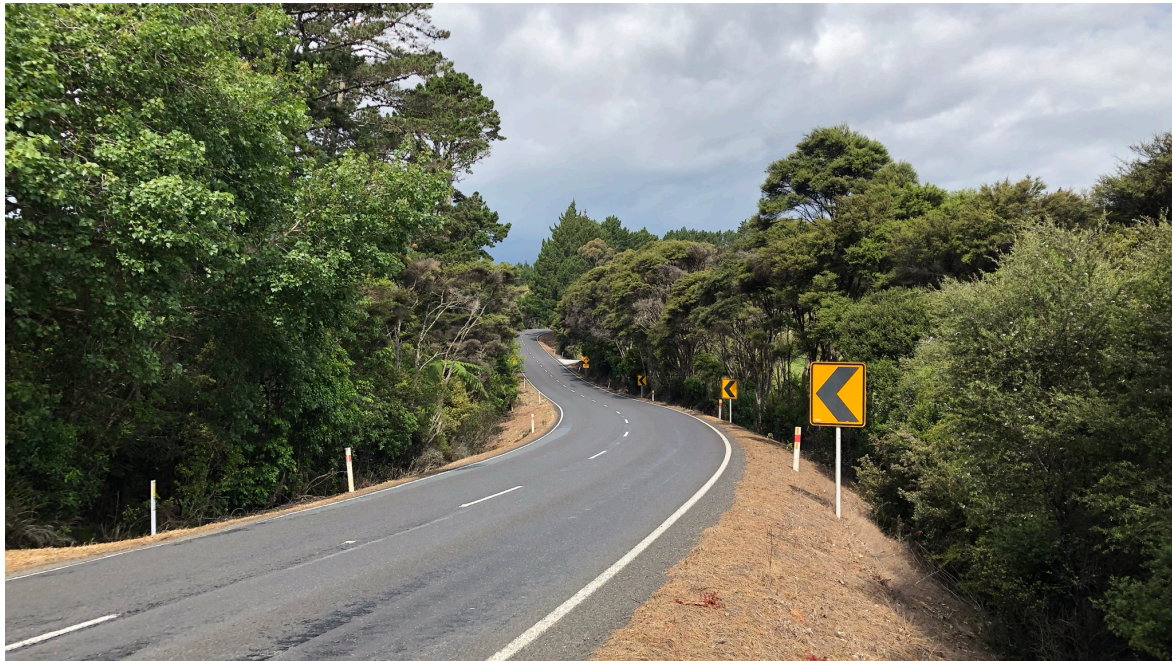
Photograph 2: Proposed Vehicle Access – Visibility to South
