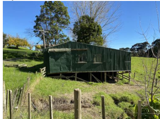
Shearing shed– location 4
