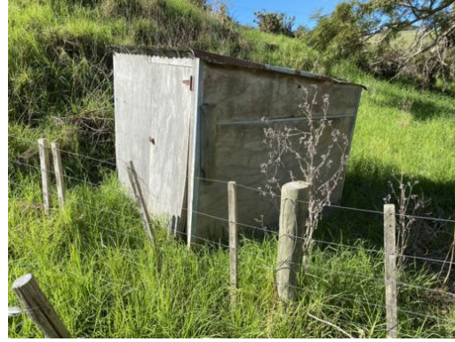
Plywood shed– location 3
