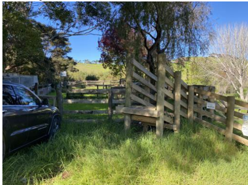
Loading ramp – location 1
