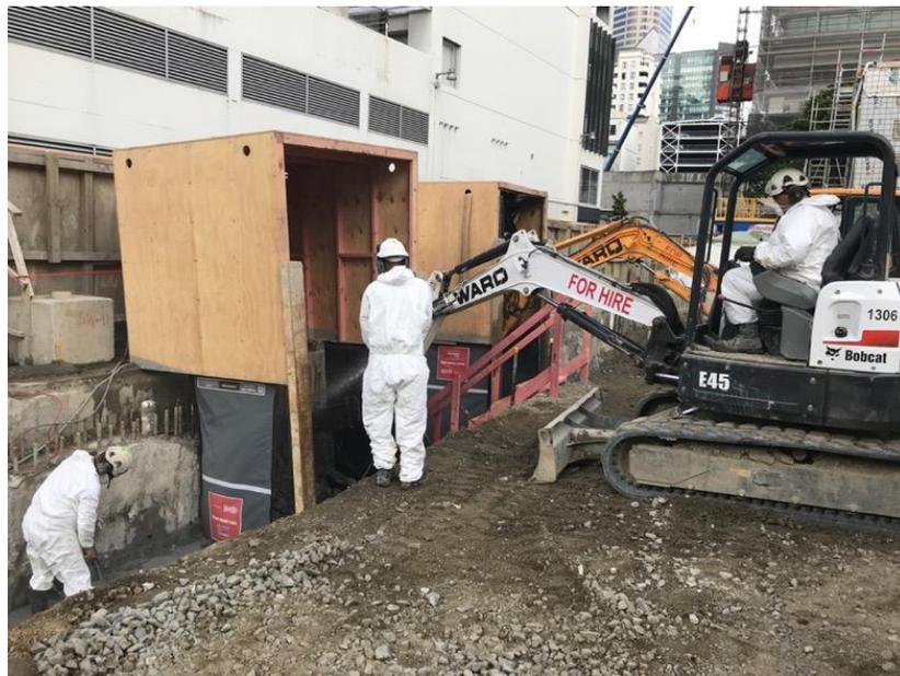
*Figure 15 - Example of a rock breaking enclosure*
