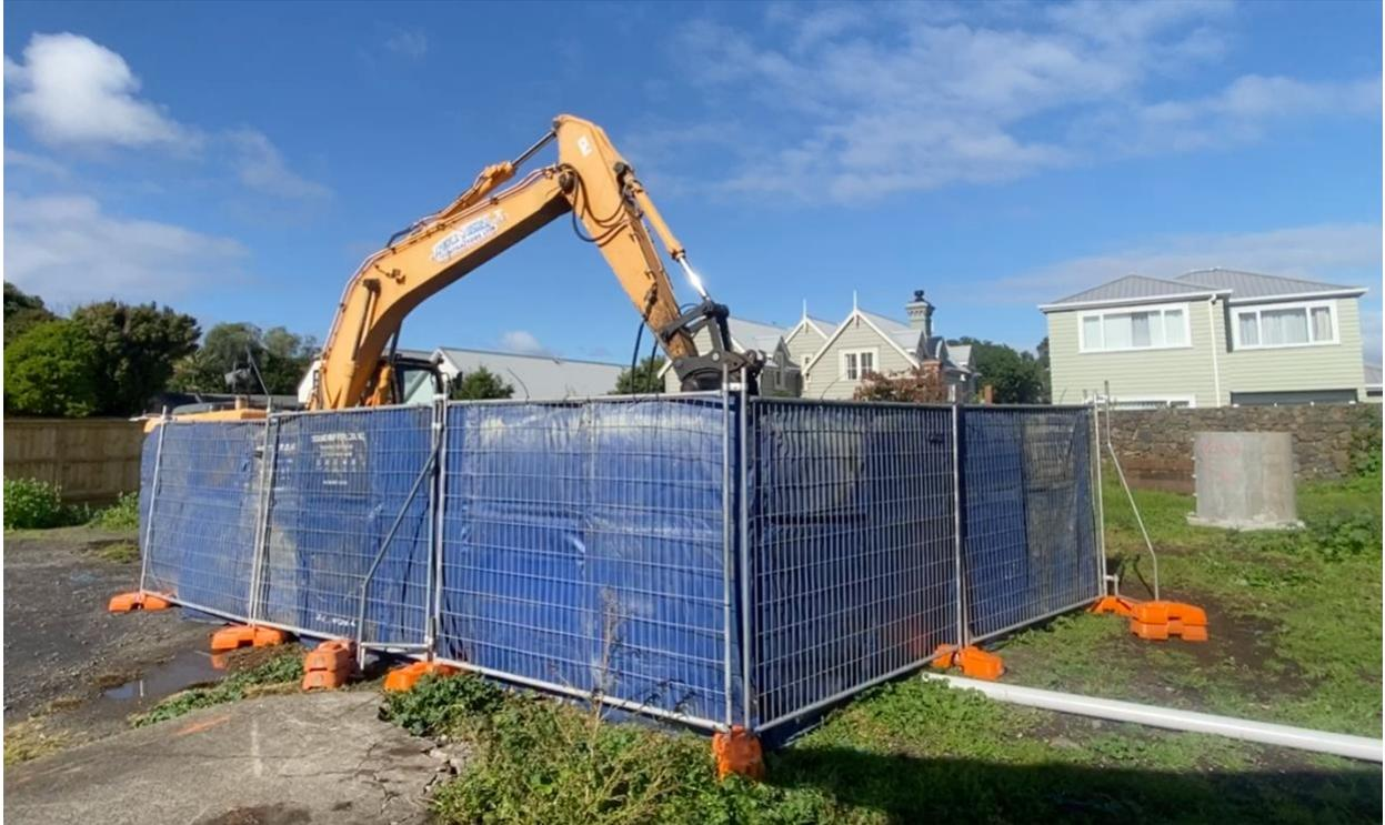
*Figure 13 - Example of Localised Acoustic blankets around area of rock breaking*
