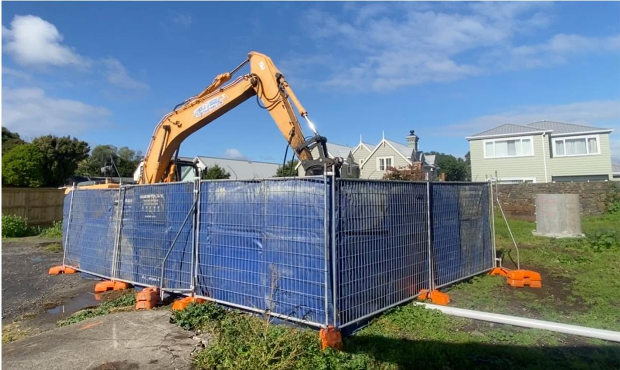
*Figure 11 - Example of Localised Acoustic blankets around area of rock breaking*
