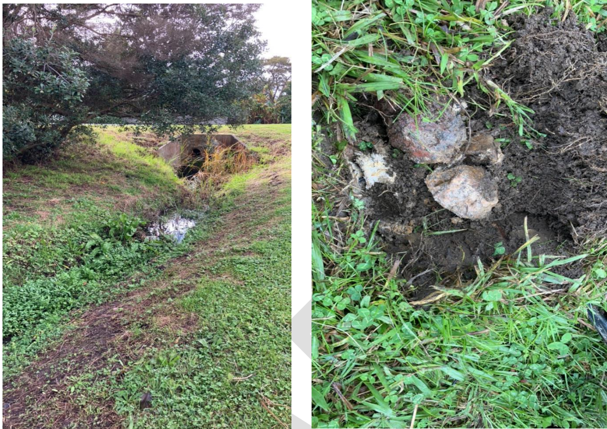
Figure 10. Site 6 looking upstream (left) where there is a doubled perched culvert, and the results of the soil plot (right).
