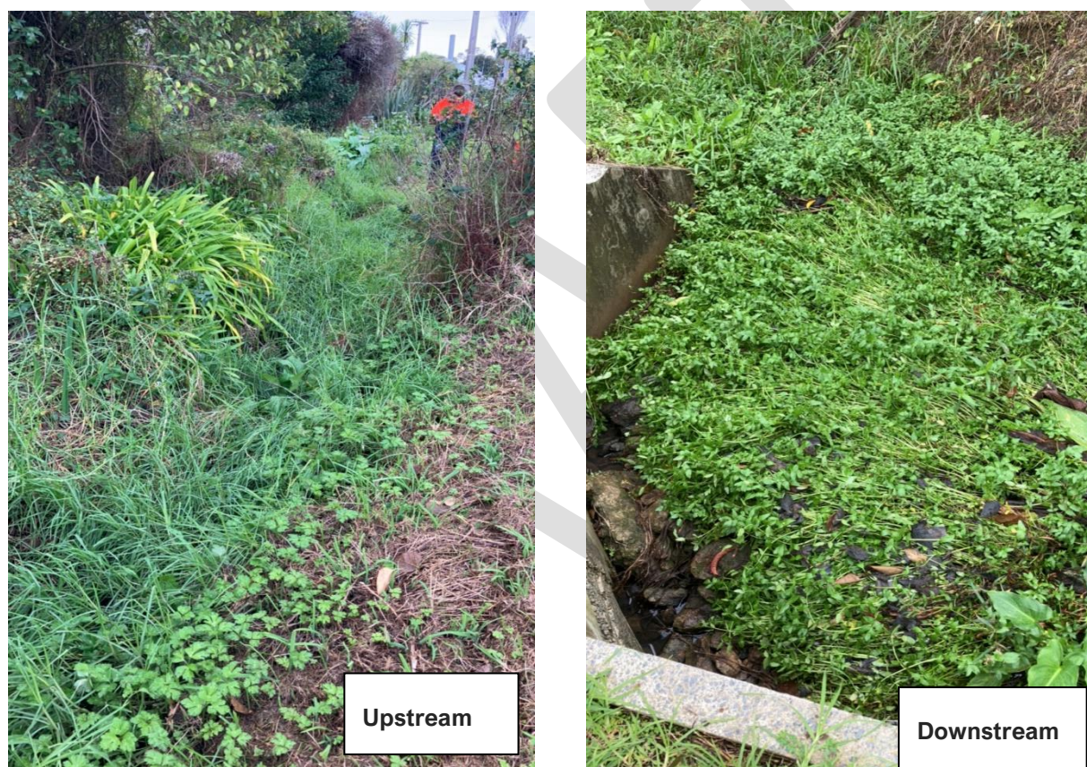
Figure 11. Site 7 with overgrowth of kikuyu within the “channel” (left), and the overgrowth of watercress at the entrance of the blocked culvert (right).
