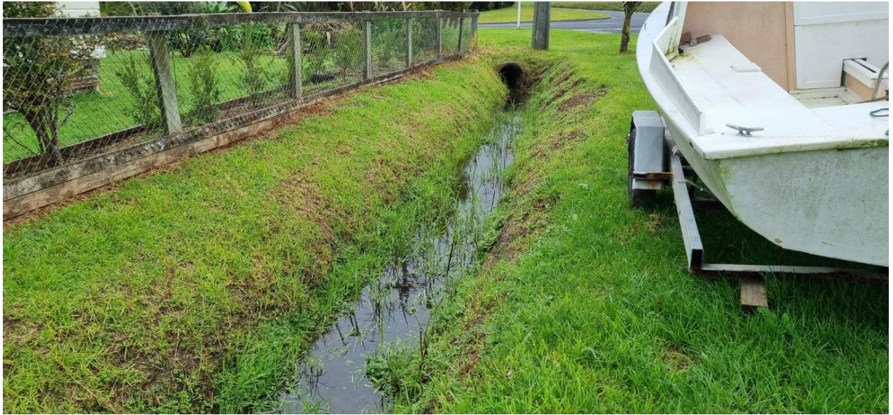
Figure 30. Existing cut swale drain along Nikau Road
