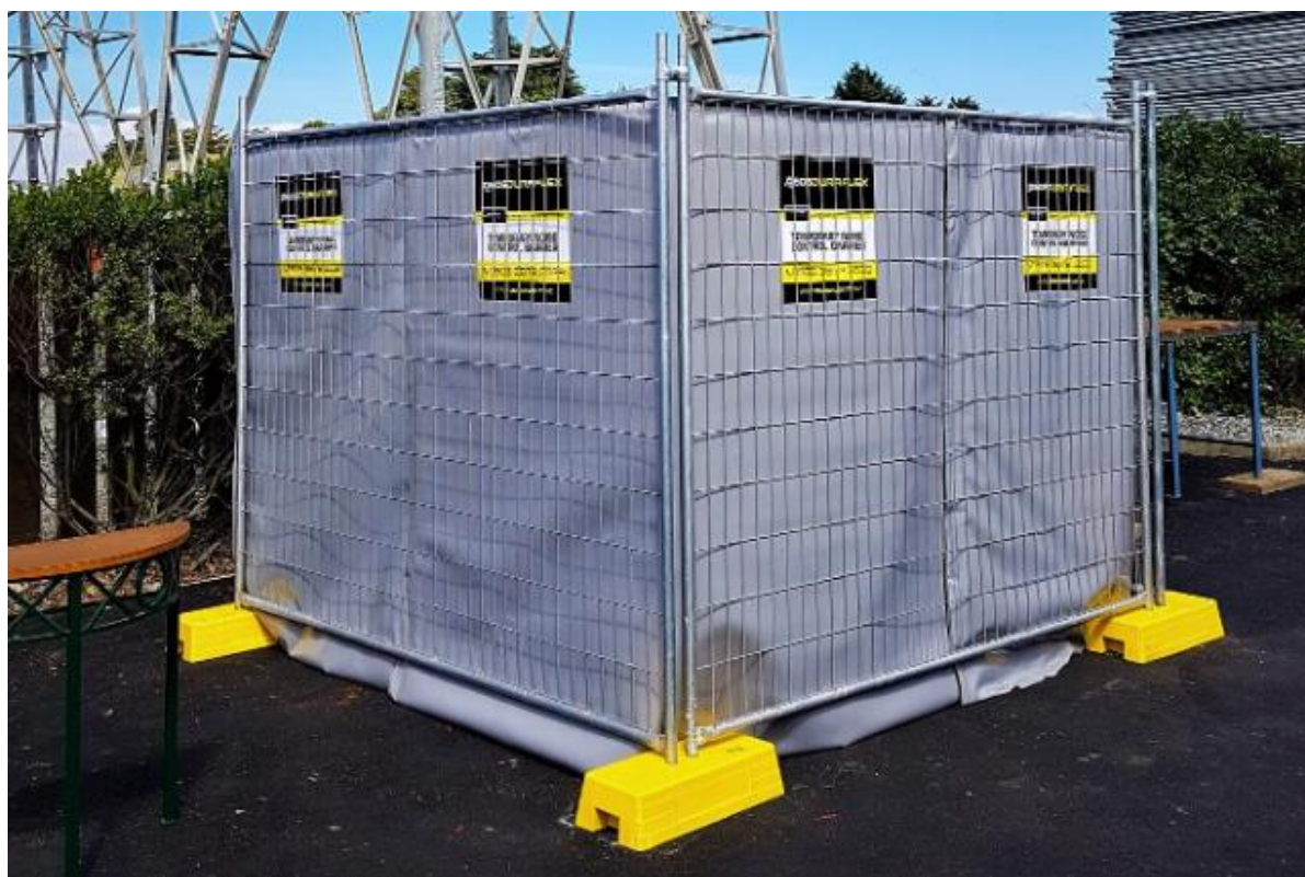
Figure 10 Example Setup of Acoustic Shroud Around Breaker Attachment
