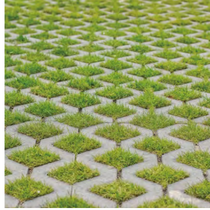
BIN COLLECTION AREA - GRASS BLOCKS
