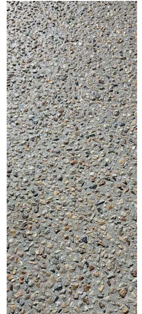
DRIVEWAYS - CONCRETE WITH CREAM AGGREGATE/OXIDE, LIGHT EXPOSED FINISH
