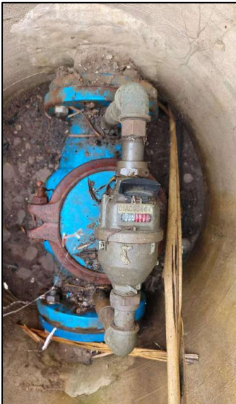
Figure7: Existing meter and backflow preventer for fire sprinkler
