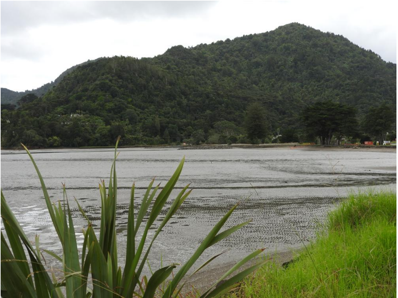
Figure 2-1: The iconic Huia Bay with recently constructed groynes and seawall protected the Huia Domain foreshore in the background
