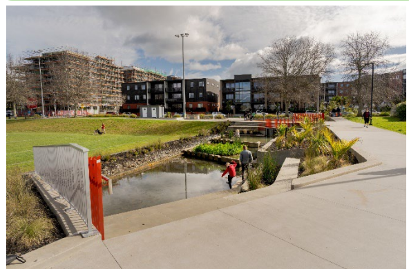
Te Kaitaka / Greenslade Reserve sports park was lowered, and a wetland constructed to better manage stormwater. Image credit: Eke Panuku, Te Ara Awataha.
