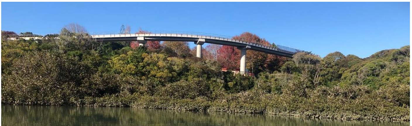
New rail bridge. Image credit: NZTA.
