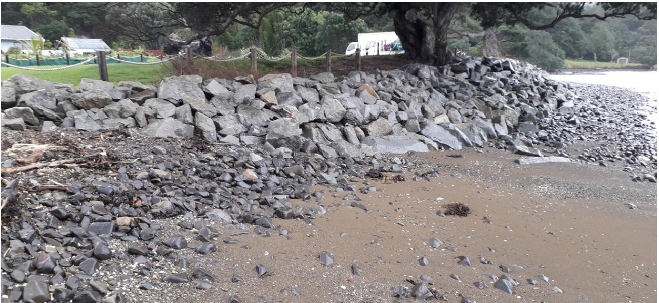
Figure 4: Private rock revetment protecting the Motairehe urupā
