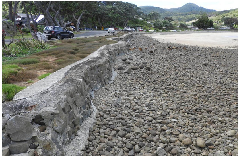
Mulberry grove seawall, with salt tolerant vegetation behind seawall crest.
