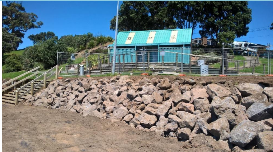
Mellons Bay rock revetment during construction 2018 (Source: Auckland Council)
