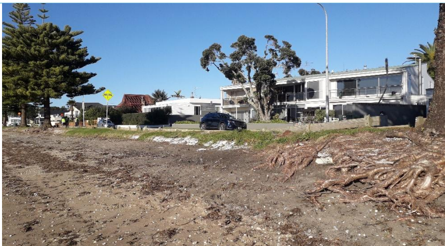
Sandbags placed as backstop protection along The Parade, northern Eastern Beach (Source: Auckland Council)
