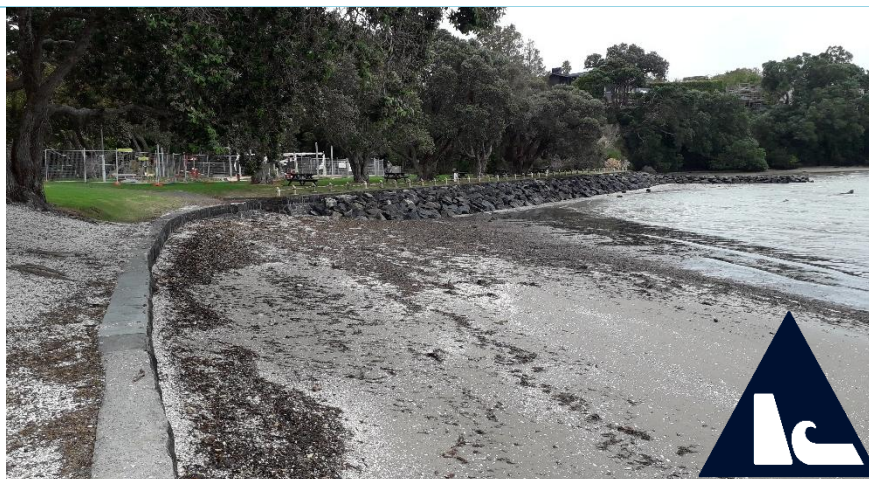
Concrete seawall and rock toe protection at Cockle Bay (Source: Auckland Council)
