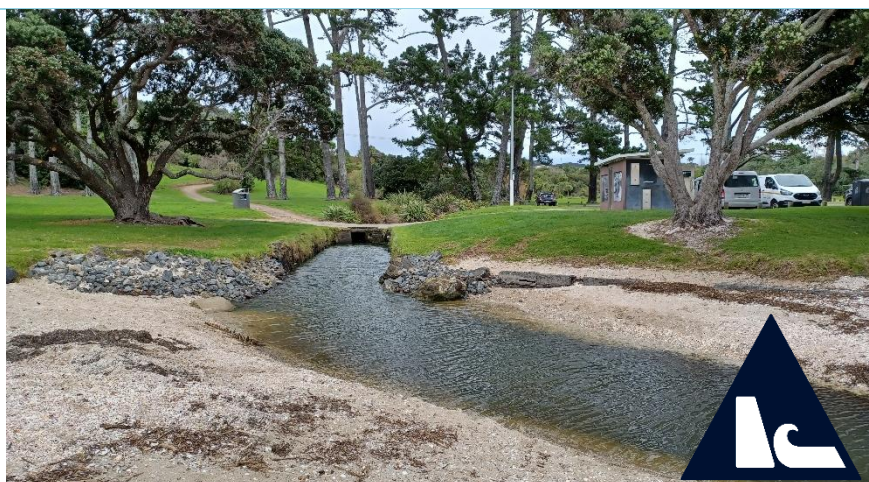
Stream training walls: southern end of Eastern Beach (Source: Auckland Council)
