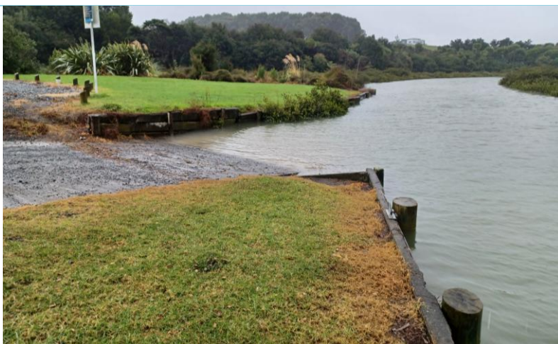
Timber retaining walls, Whitford boat ramp (Source: Auckland Council)
