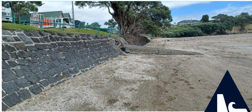
Masonry seawall at Howick Beach (Source: Auckland Council)
