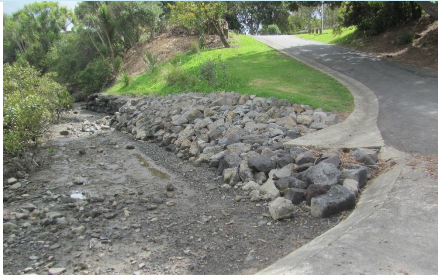
Stacked rock armouring Tiraumea ramp access. Source: Auckland Council
