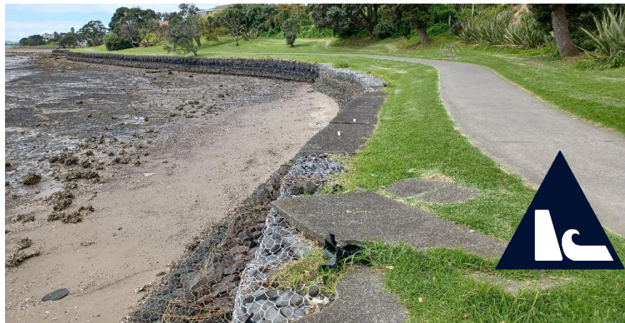
Rotary walkway along Fisher Parade Esplanade Reserve, armoured with stacked gabion basket seawalls (Source: Auckland Council)
