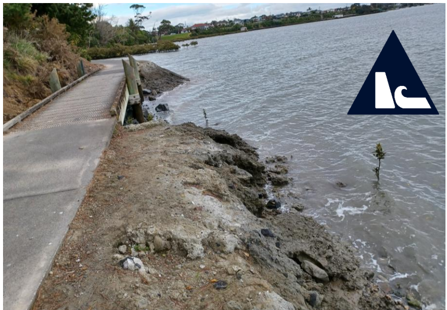
Mudcrete armoured of Rotary walkway section near St Kentigern College with boardwalk section bridging ignimbrite exposure (Source: Auckland Council)
