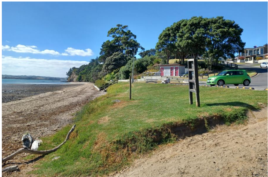
2025 Mellons Bay rock revetment with established grass cover (Source: Auckland Council)
