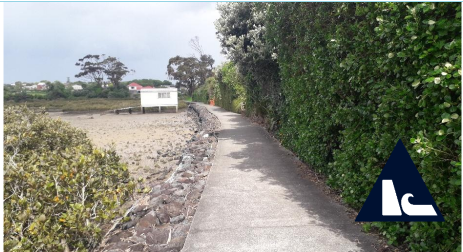
Rotary walkway along Tāmaki Bay Drive Reserve armoured with stacked gabion basket seawall with rock capping (Source: Auckland Council)
