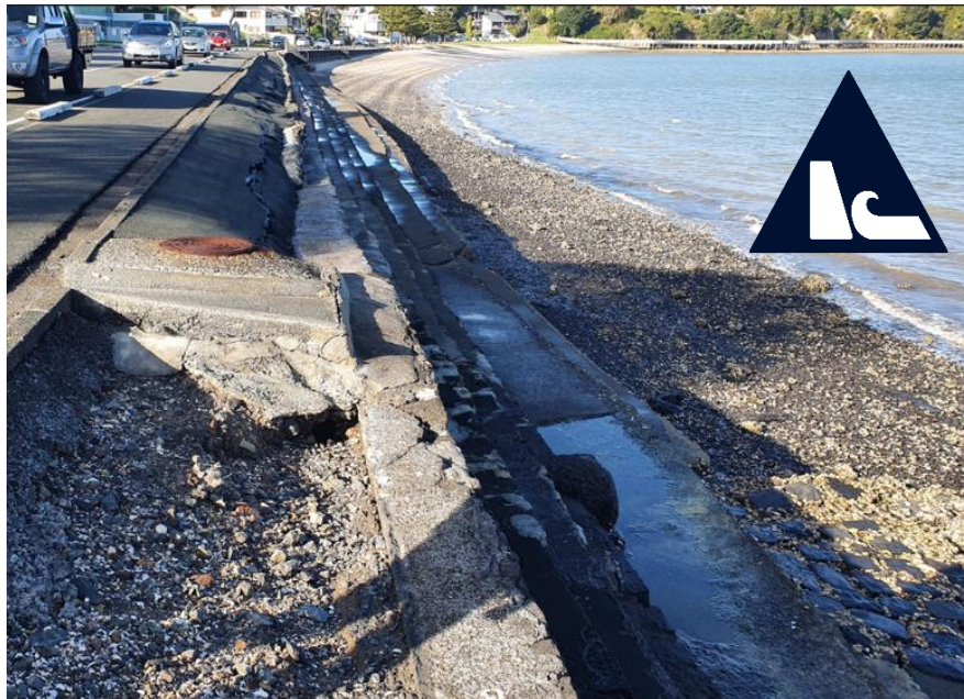
Seawall at Little Bucklands Beach, Auckland Transport asset (Source: Auckland Council)
