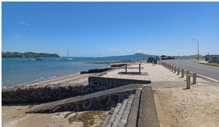
Stepped masonry wall and groyne field at the northern end of Bucklands Beach (Source: Auckland Council)
