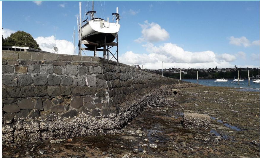
Granger Point masonry seawall (Source: Auckland Council)
