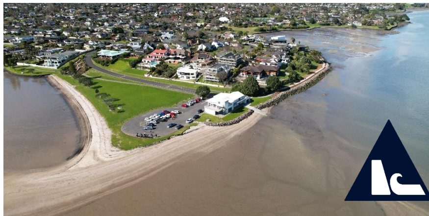
Bramley Drive Reserve rock revetment armouring Rotary walkway and Pakuranga Sailing Club building with natural sandspit fronting the low reclaimed grass reserve at the entrance to Waka Aranga Creek (Source: Auckland Council)
