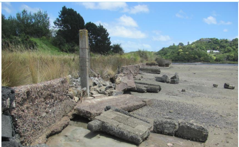
Remnant structures along coastal margin of Broomfields Reserve (Source: Auckland Council)
