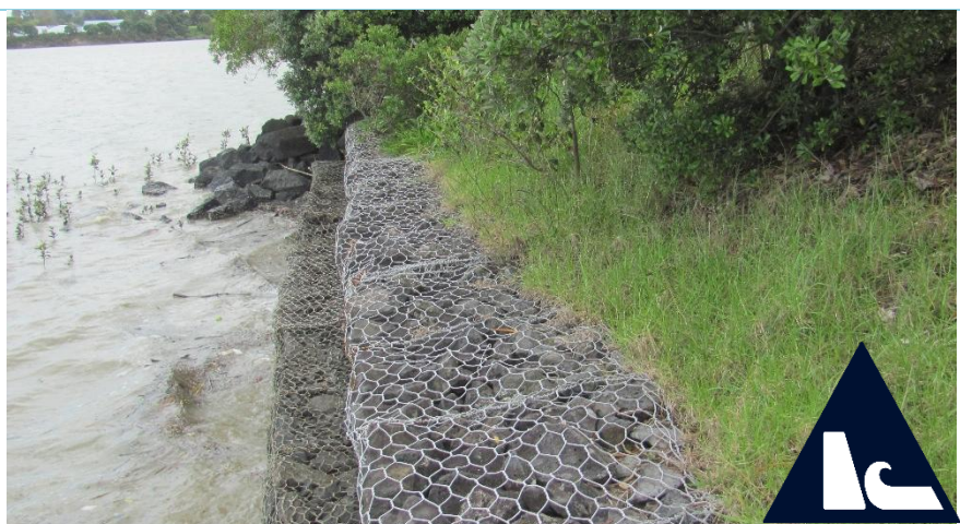
Riverina Reserve armoured with stacked gabion basket seawalls (Source: Auckland Council)
