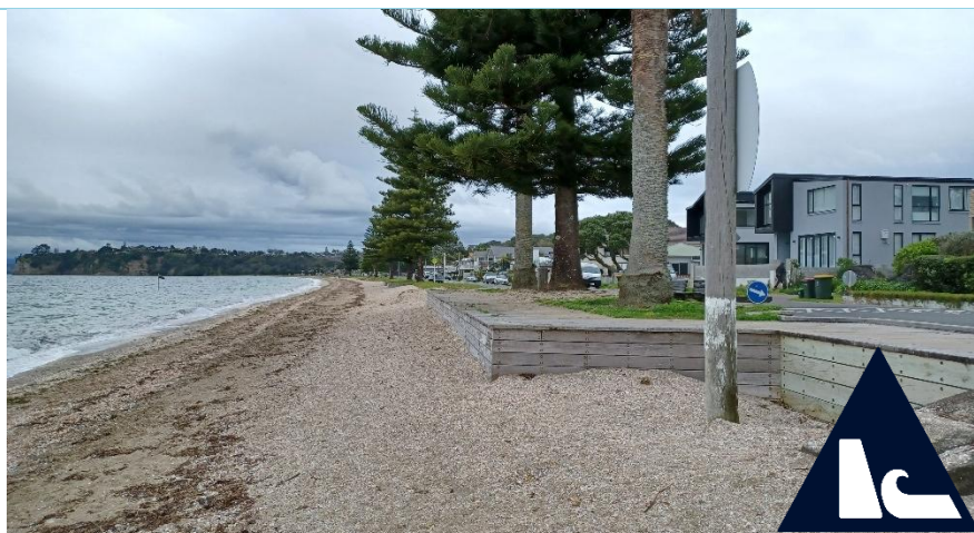
Timber backstop seawalls around trees at the northern end of Eastern Beach (Source: Auckland Council)
