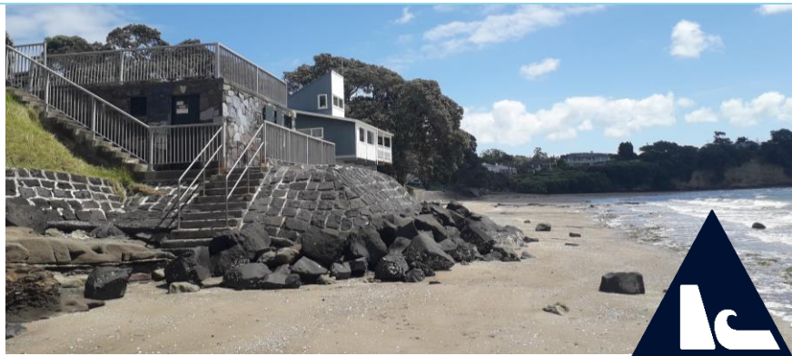
Rock revetment armouring the wastewater pumping station Howick Beach (Source: Auckland Council)
