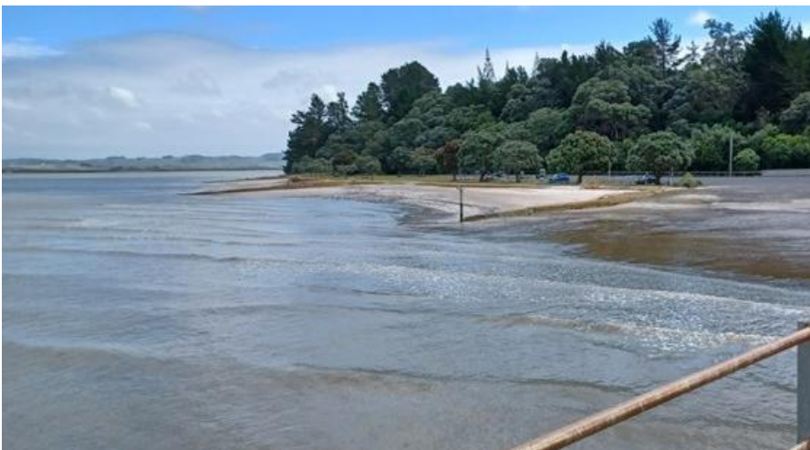
Figure 4: Shelly Beach Reserve seen from the wharf, with three groynes and seawall
