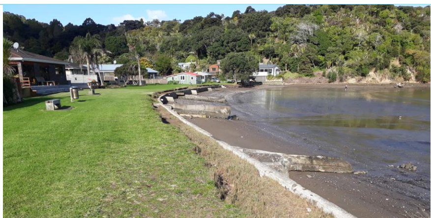
Seawall and associated coastal structures (abutments and stormwater outfalls) protecting the reclaimed edge of Foster Bay Reserve (Source: Auckland Council)
