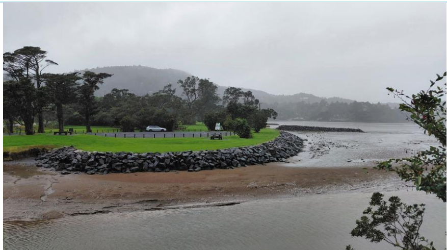
Rock revetment to the west of Huia Domain extending into Huia Stream (Source: Auckland Council)
