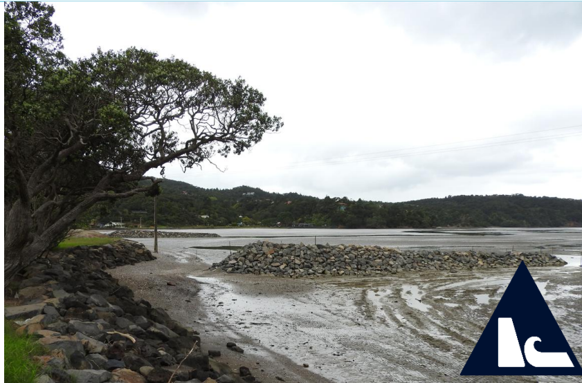
Recently completed detached rock groynes and sand replenishment at Huia Domain (Source: Auckland Council, 2018)
