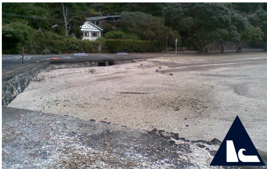
French Bay – low grouted seawall armouring Otitori Bay Road.
