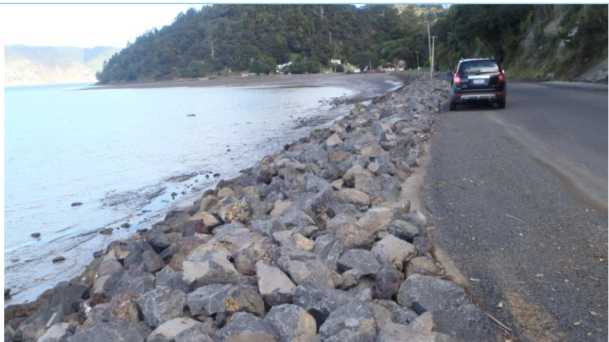
Rock revetment protection the edge of more exposed sections of Huia Road (Source: Auckland Council)
