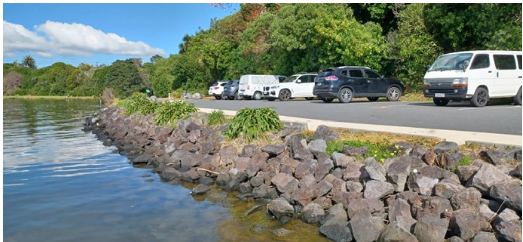
Rock armoring of carparking area, Ōrākei Basin (Source: Auckland Council)
