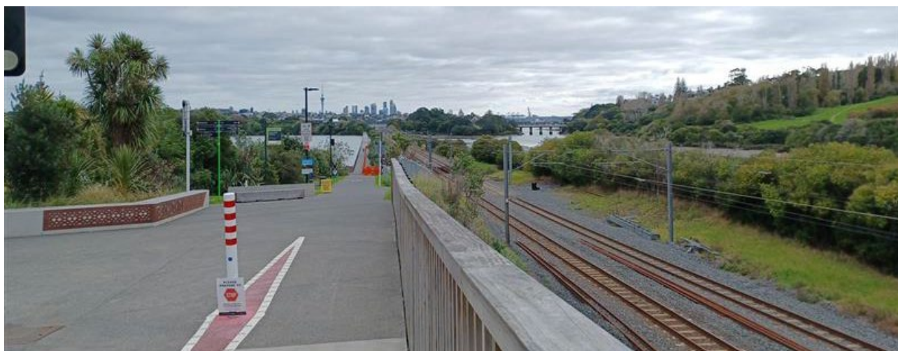
Figure 4: View north west toward the central business district along the shared path and rail corridor. Source: Auckland Council 2025
