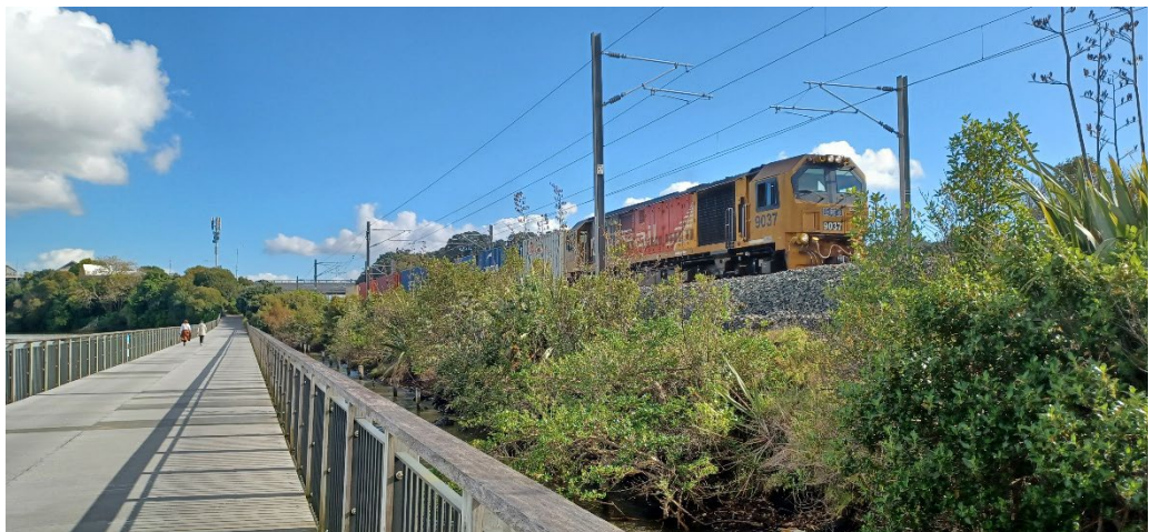
Armoured railway embankment and boardwalk, Ōrākei Basin (Source: Auckland Council)
