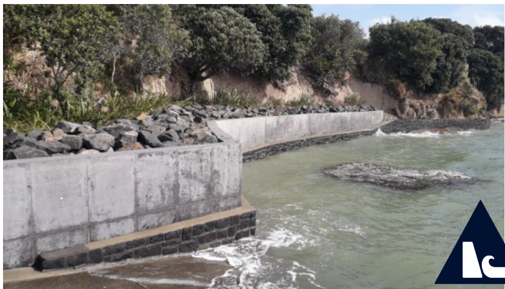
Andersons Bay seawall (Source: Auckland Council)
