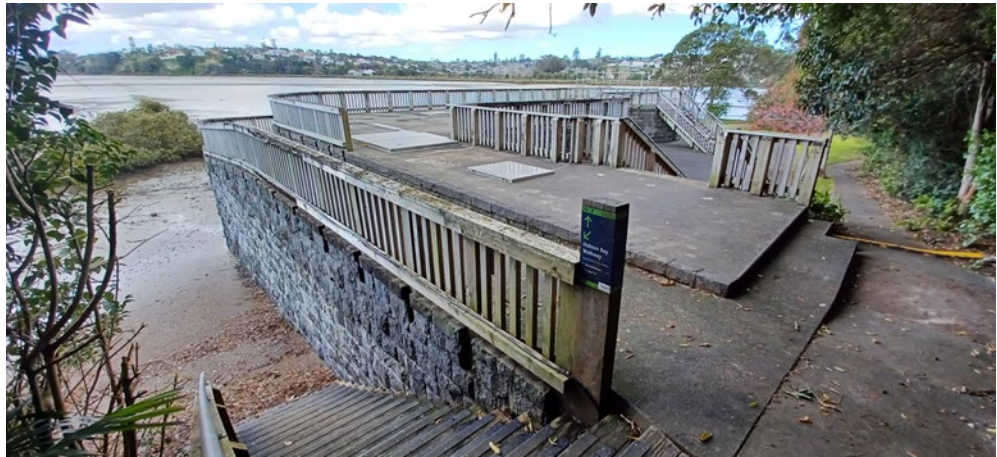
Logan Terrace wastewater pumping station (Source: Auckland Council)
