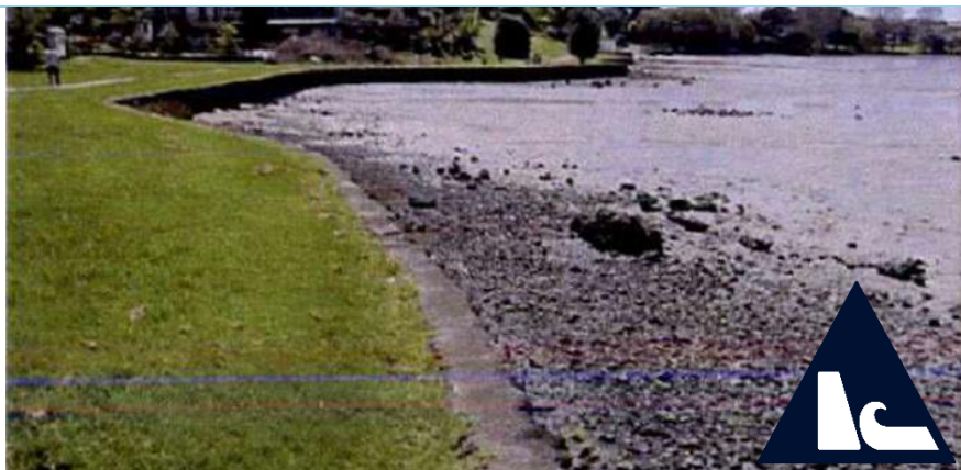
Panmure Basin walkway and basin perimeter armoured with rock masonry seawall (Source: Auckland Council)
