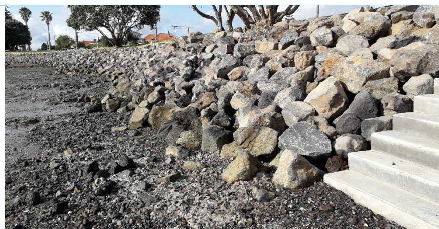
Dunkirk Reserve section of rock revetment armouring. Source: Auckland Council
