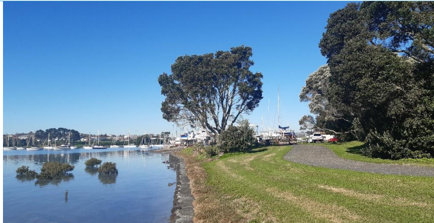
Low masonry seawall armouring Mount Wellington War Memorial Reserve. Source: Auckland Council
