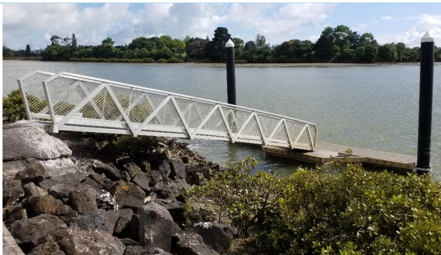
Flat Rock reserve edged with tipped rock armour. Source: Auckland Council
