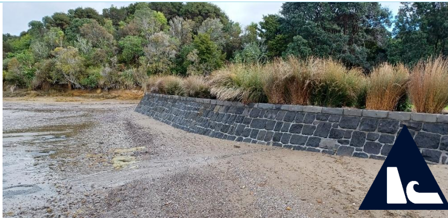
Tahaki Road end cul-de-sac armoured with masonry seawall (foreground) with densely vegetated margin along Wai-o-Taiki Nature Reserve (background) (Source: Auckland Council)
