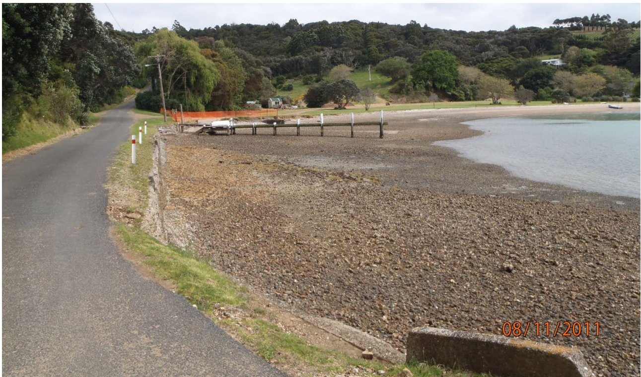
West along Anzac Road, road access to Orapiu Wharf, with coastal armouring along the road edge and private jetty structure in the mid view. Source Auckland Council 2011
