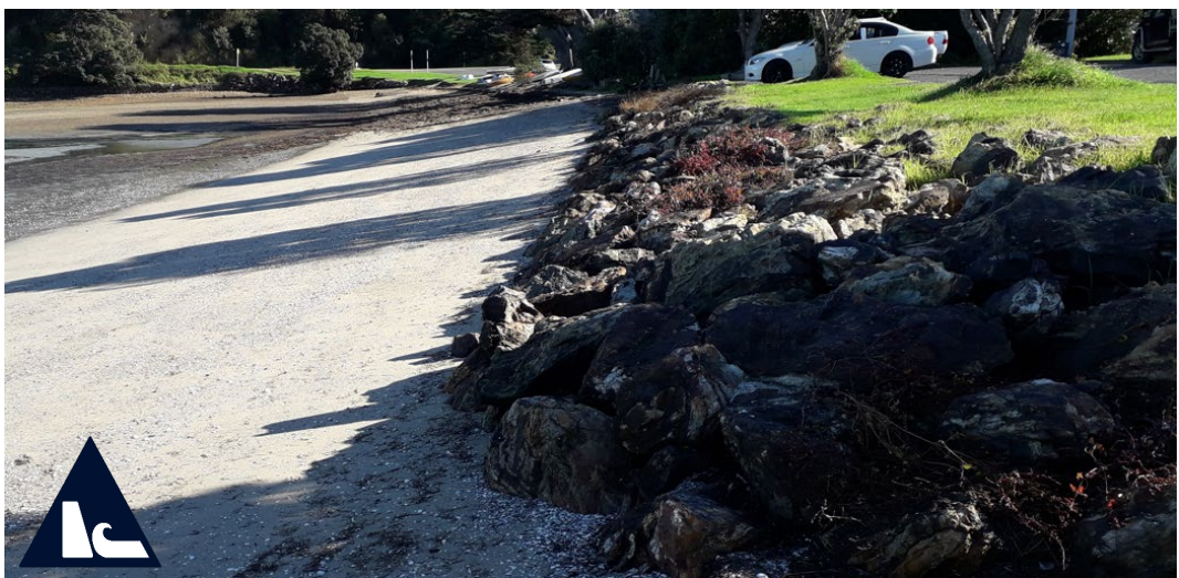
Rock revetment armouring at Surfdale Beach.
