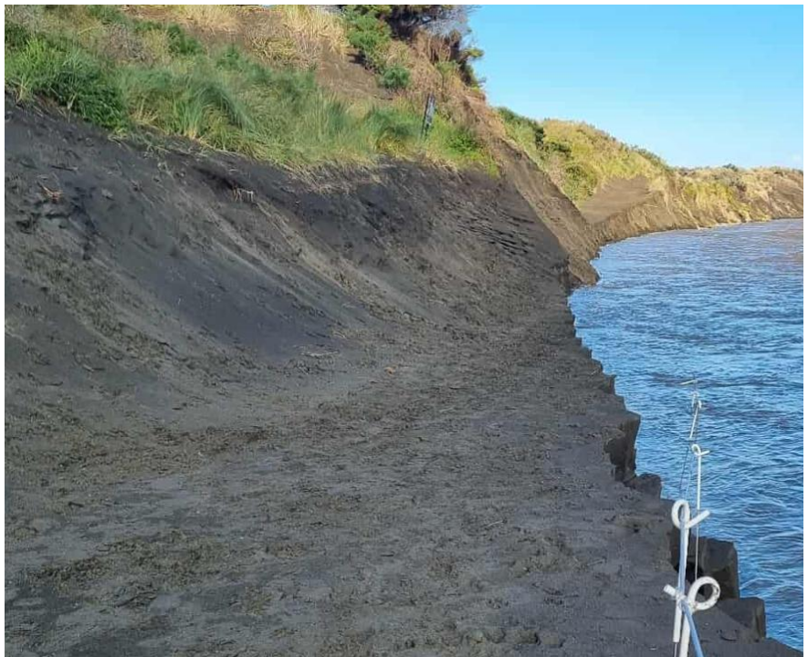
Restricted beach access following heavy rainfall (Source: Auckland Council)
