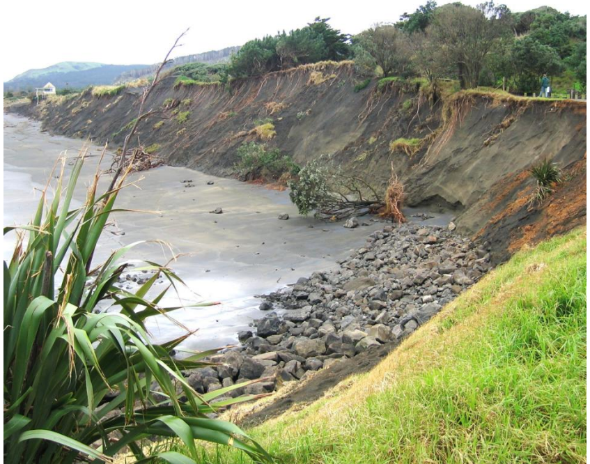
Erosion at the southern end of Muriwai Beach (Auckland Council, 2008)
