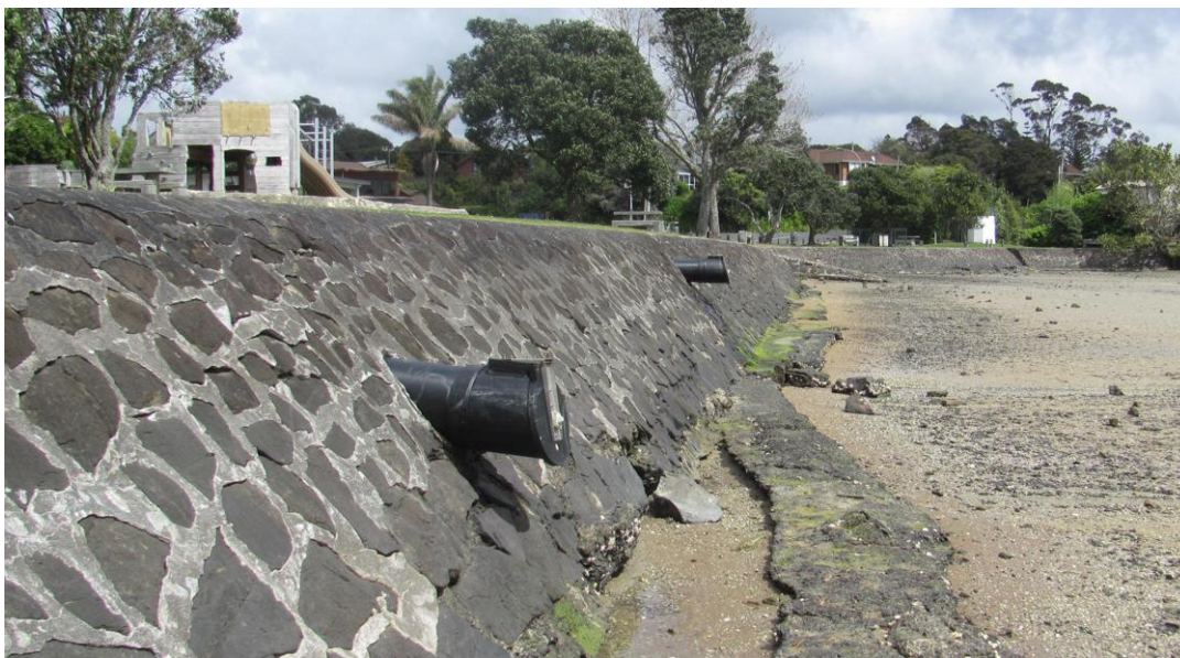
Rock masonry seawall, Christmas Beach, Herald Island (Source: Auckland Council)
