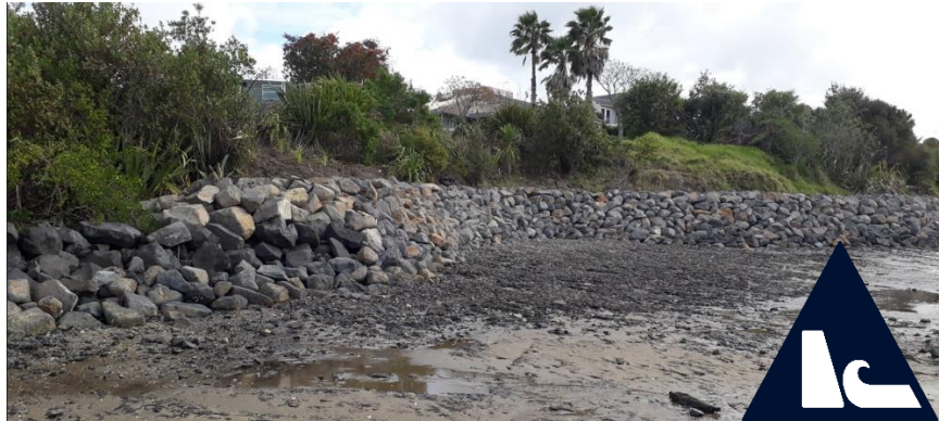
Rock revetment seawall, Spinnaker Strand (Source: Auckland Council)
