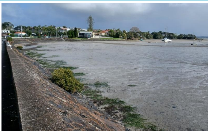
Sloped masonry seawall armoured West End Road, Cox's Bay (Source: Auckland Council)
