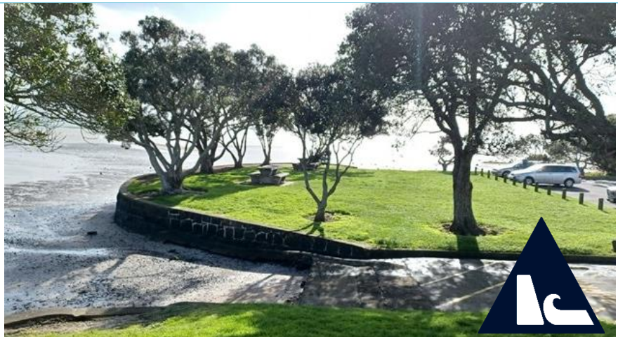
Eric Armishaw Reserve armouring with masonry seawalls (Source: Auckland Council)
