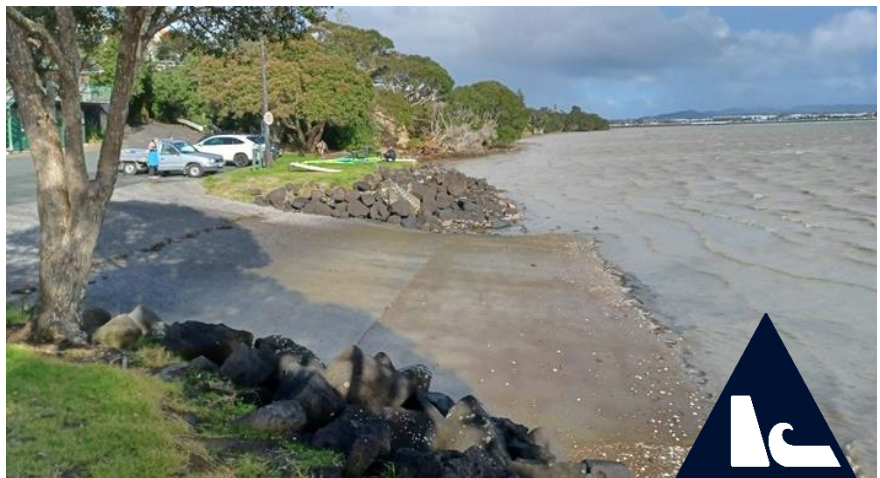
Rock revetment adjacent to the southern boat ramp at Raymond Reserve (Source: Auckland Council)
