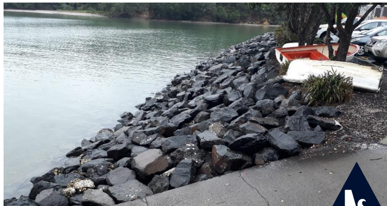
Island Bay dinghy ramp and rock revetment armouring edge of car park. (Source: Auckland Council)
