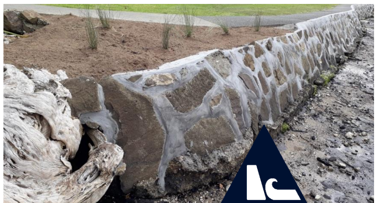
Taipari Strand grouted rock seawall and concrete footpath capping (Source: Auckland Council)
