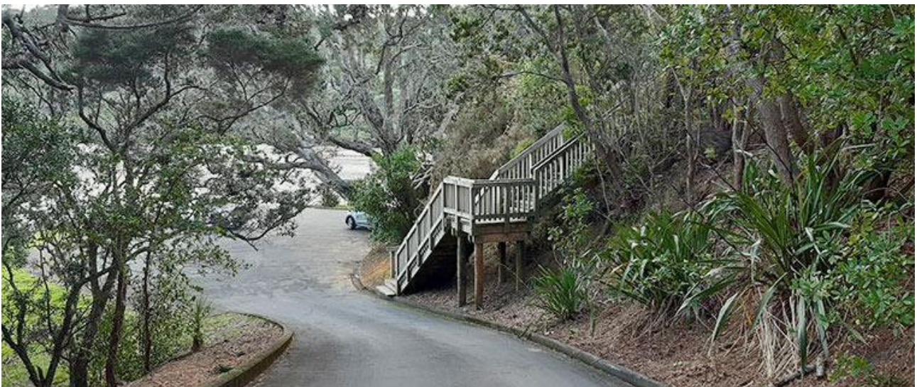
Maukau Reserve accessway leading to the boat ramp area (source Auckland Council)
