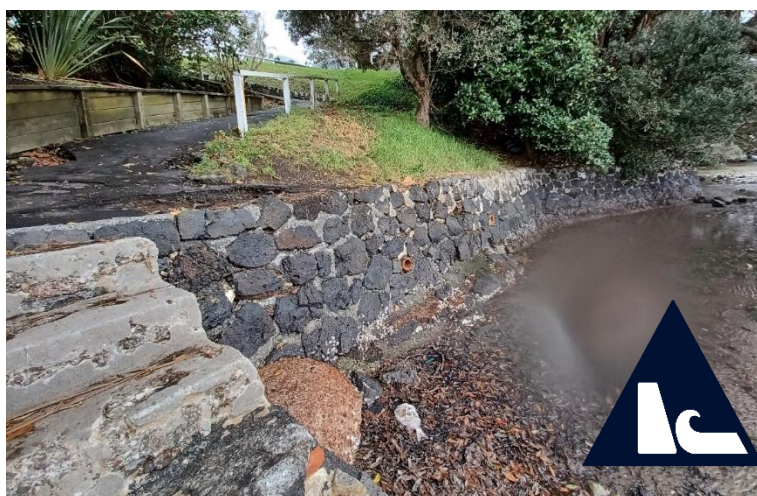
Sloped masonry seawall armoured West End Road, Cox's Bay (Source: Auckland Council)
