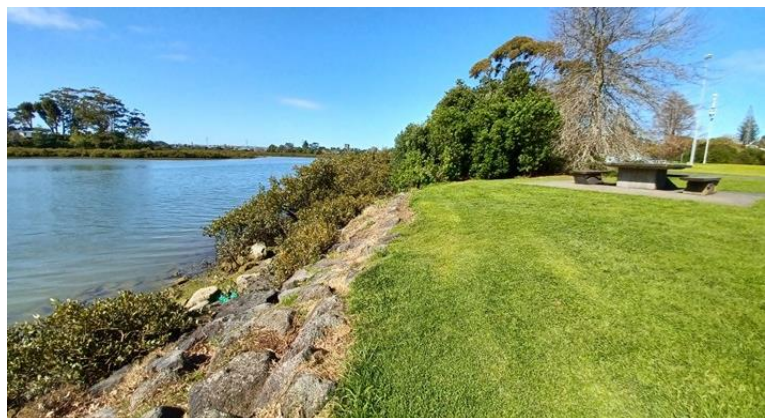
a) Concrete seawall and b) tipped rock armouring, Archibald Park (Source: Auckland Council)
