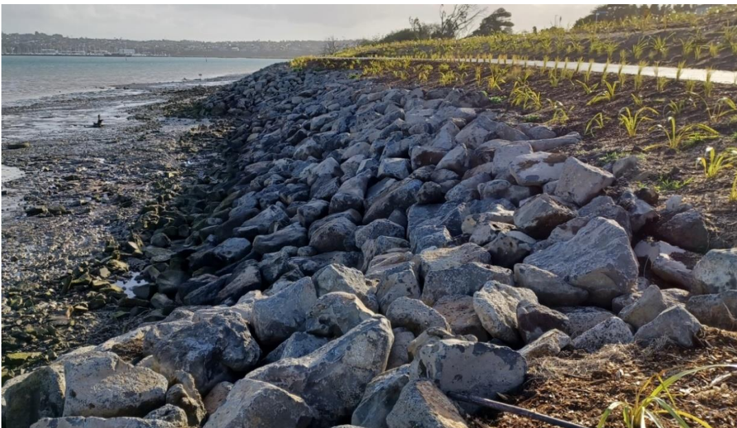
Figure 1-2: Rock revetment armouring and coastal path, Scott Road (Source: Auckland Council)
