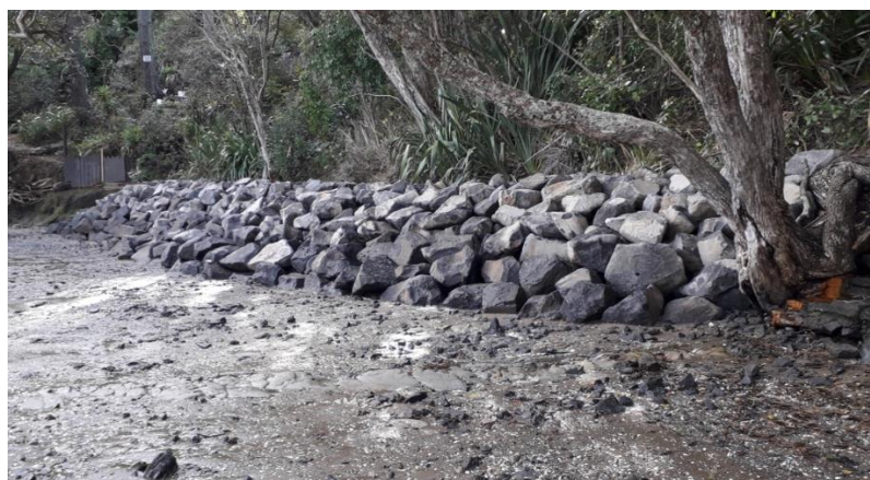
Rosecamp Road Reserve rock revetment armoring at northern end of the reserve. (Source: Auckland Council)
