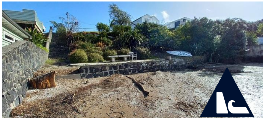
Johnstone Road Reserve seawall and steps (Source: Auckland Council)
