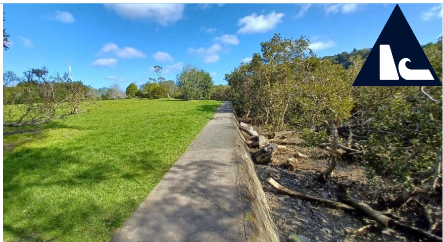
Taipari Strand grouted rock seawall and concrete footpath capping (Source: Auckland Council)
