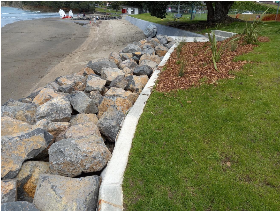
Figure 10: Renewed rock revetment and shotcrete seawall upgrade, Waiake Beach Reserve
