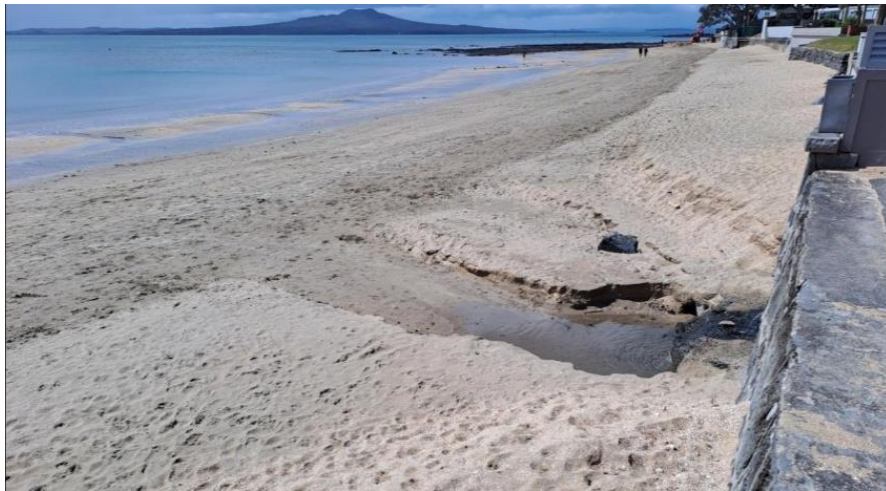
Figure 17: Council and private seawalls, stormwater outfall, and basalt intertidal reef, Milford Beach (Source: Matthew McNeil)
