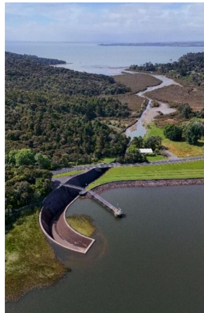
Lower Nihotupu Dam in the Waitākere Ranges.
